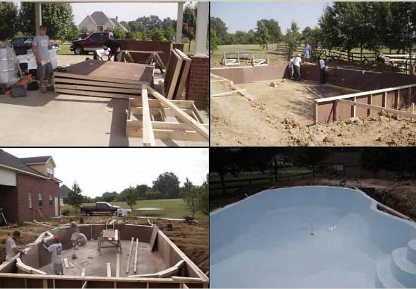
Figure 11.16: Fiberglass pool construction on site (Korekote, 2012:online).
