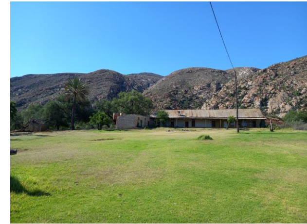
Figure 2.24: Main building on site (Author, 2022).
