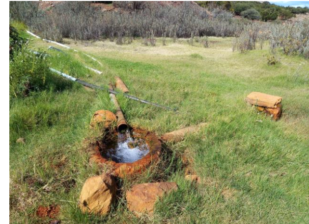
Figure 2.22: Hot water outlet (Author, 2022).
