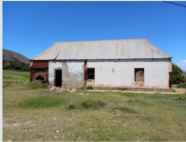
Figure 2.23: Existing building on site (Author, 2022).
