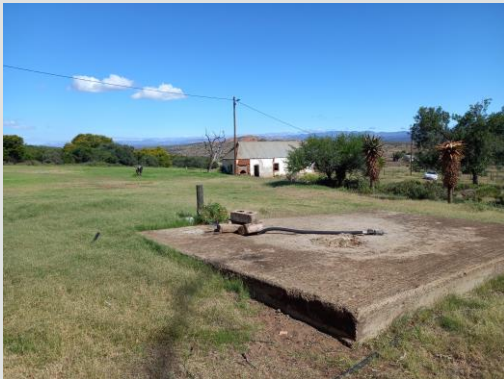
Figure 2.28: Underground water tank (Author, 2022).
