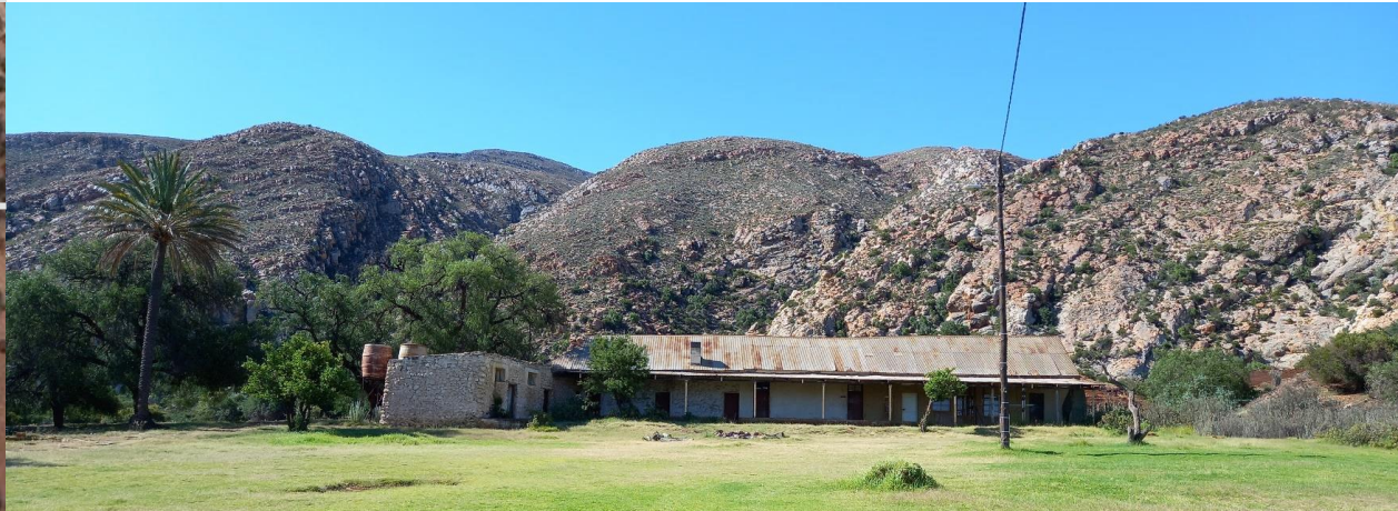
Figure 2.20: Main building on site (Author, 2022).
