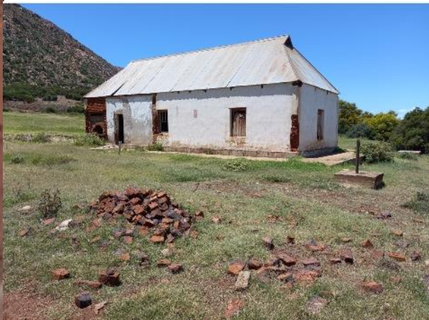
Figure 2.21: Existing building on site (Author, 2022).
