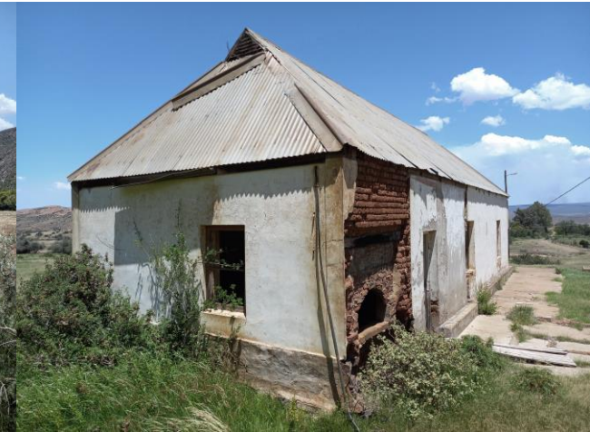
Figure 8.24: Exterior of existing building (Author, 2022).
