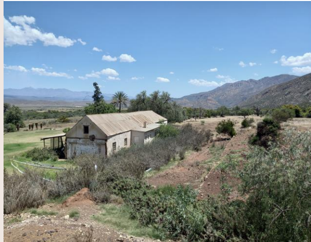
Figure 8.23: Existing building on site (Author, 2022).
