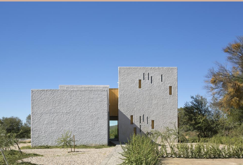
Figure 6.41: Punctured wall (Davies, 2016: online).
