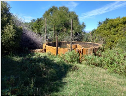
Figure 2.31: Dam on site (Author, 2022).
