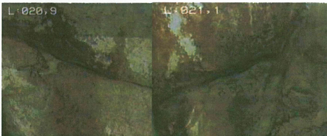
Figure 6-3 Borehole video of the fracture zone in borehole UO5 at a depth of between 20.9 – 21.1 m below surface, showing a fracture zone thickness of about 200 mm
