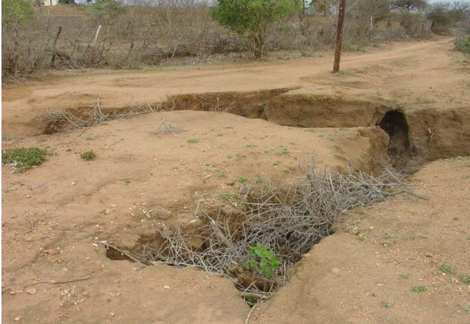
Figure 2.2 Road condition. An example of severe soil erosion that affected the road condition in the Nkonjw Chiefdom. Photo was taken by researcher.
