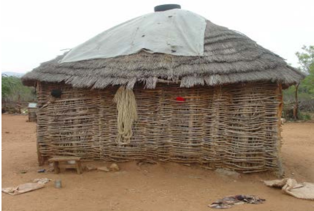
Figure 3.1 A traditionally built structure/room. Its framework is made up of interlaced sticks that usually are plastered with special mud.
