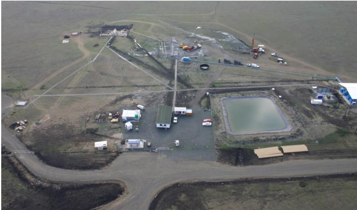
Figure 2-10 An aerial view of the Majuba UCG pilot plant, adapted from (Perashad et al., 2018a)
