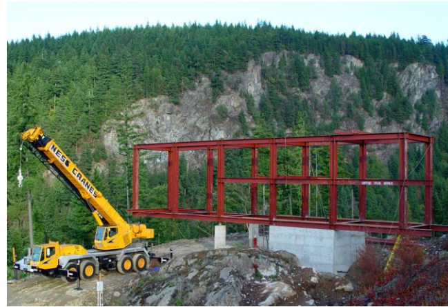
Figure 6.26: Steel framework (Anderson,2010).
