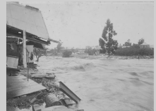
Figure 2.19: Flooded East Burger Street (du Plessis,2020:online)
