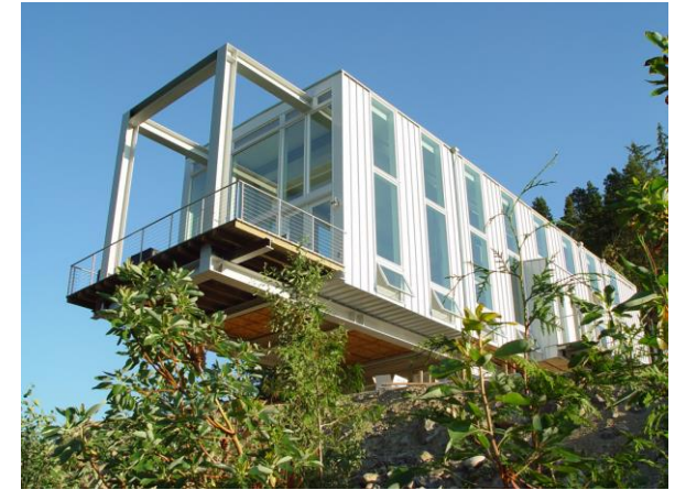
Figure 6.27: Cantilever on site fully paneled (Anderson,2010).
