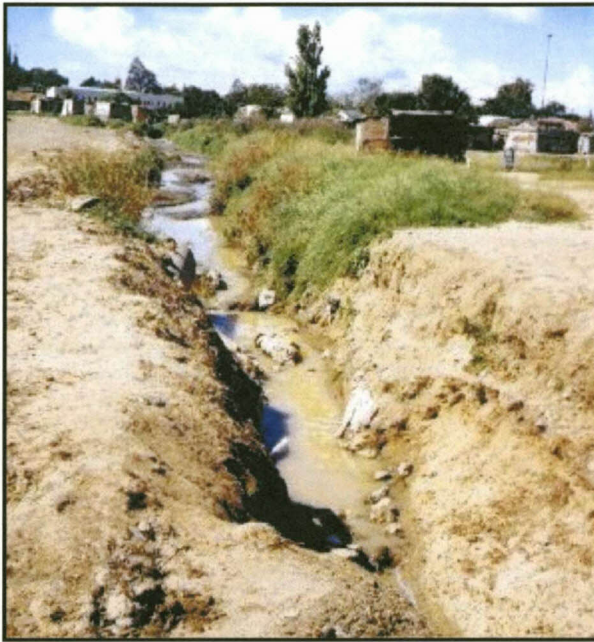
Photograph 5.2 Drainage from Bochabela residential section
