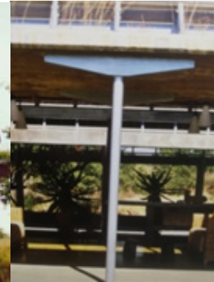
Figure 261: Steel column Lengau Lodge (Venter, 2014: online).
