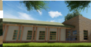
Figure 135: Exterior of social hall (Author, 2021).
