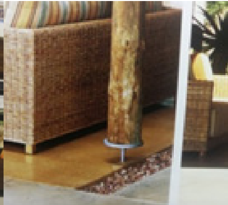
Figure 262: Gum pole column Lengau Lodge (Venter, 2014: online).
