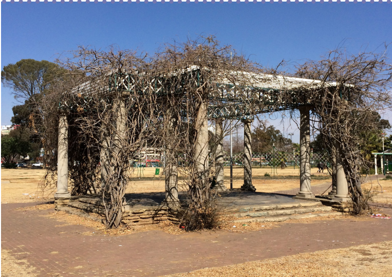
Figure 35 Pergolas on site(Author, 2019)
