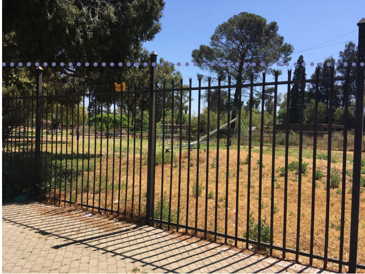
Figure 68 Restricting fence (Auhor, 2019)
