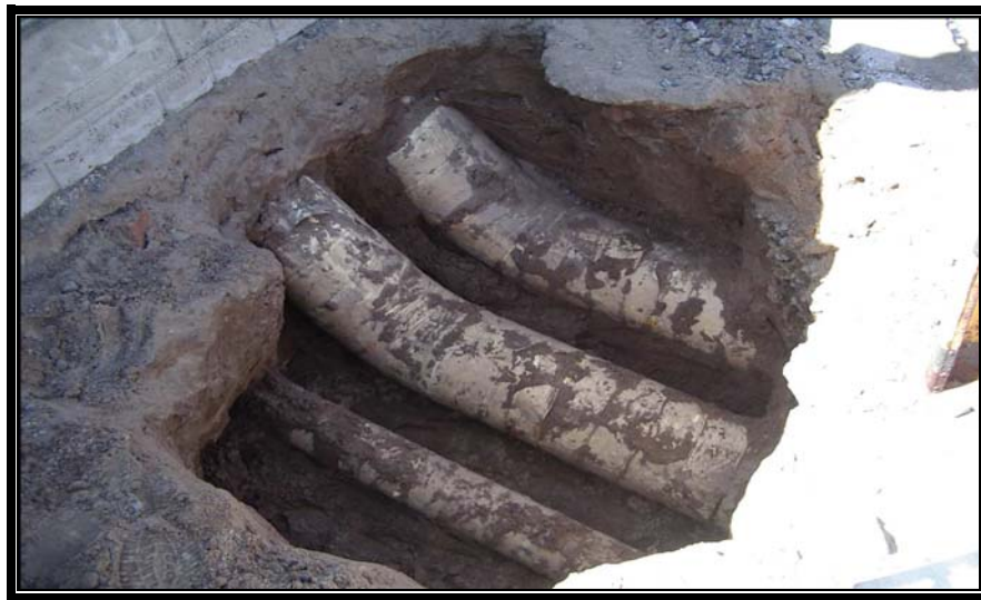
Figure 4.1 No products found around exposed fuel piping (Du Plooy 2007).
