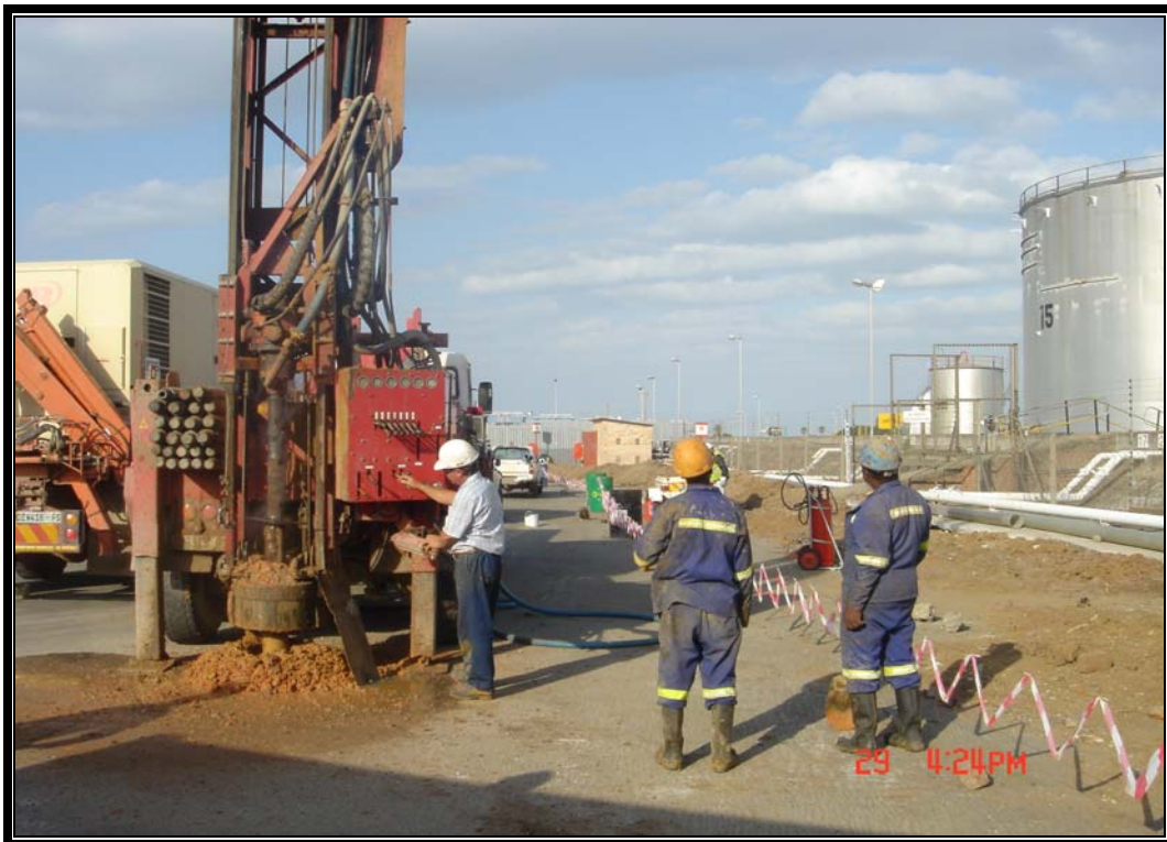
Figure 6.13 Drilling of borehole BPD1 (Usher et al. , 2009).
