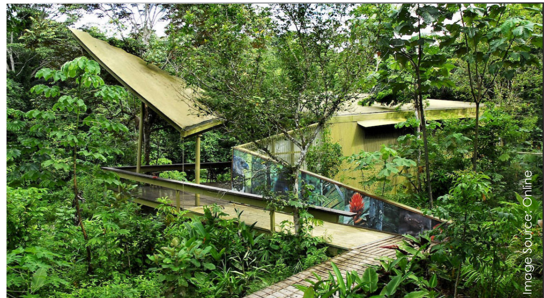
ENSITU Architects. Panarama Rainforest Discovery Centre. Cocle, Panama. Photographs: Patrick Dillion. 2012
