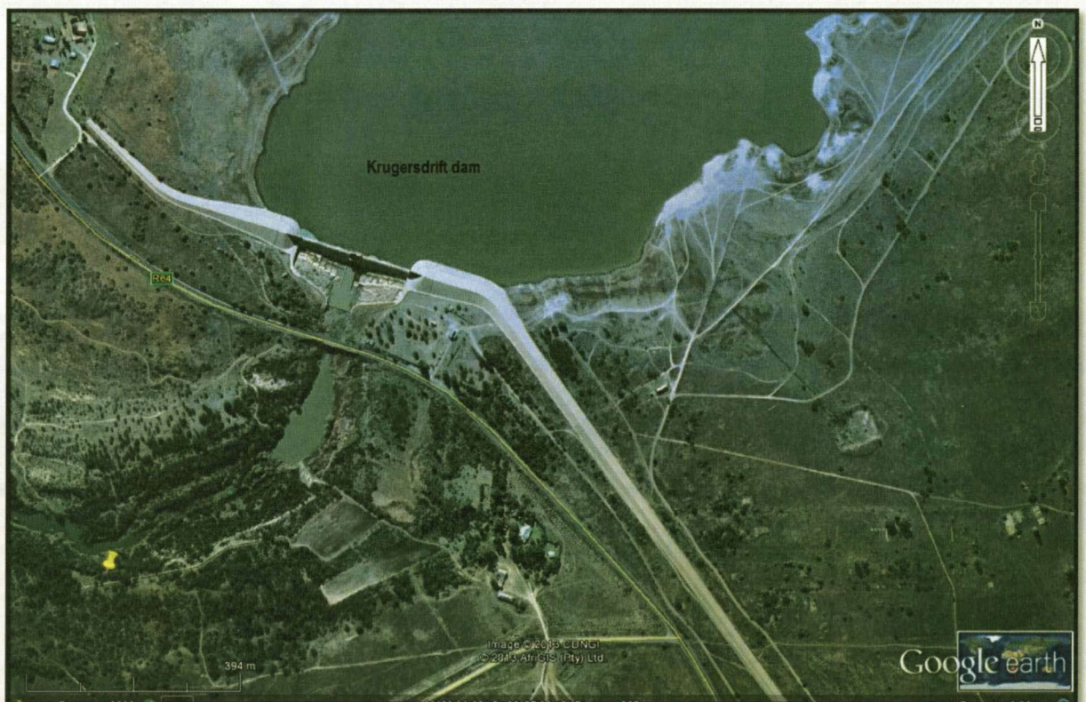
Figure 100: Krugersdrift dam (Google Earth, 2013)
