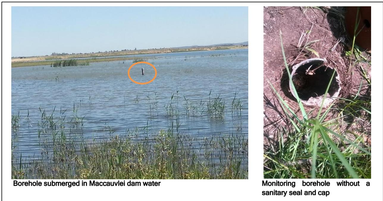
Figure 2.14: Photo showing condition of some of the monitoring boreholes.
