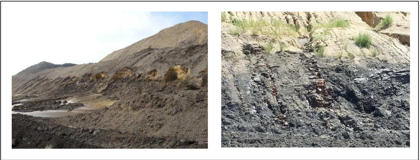
**Figure 2.19: Seepage from the interface between the hard overburden and shallow alluvium sand**
