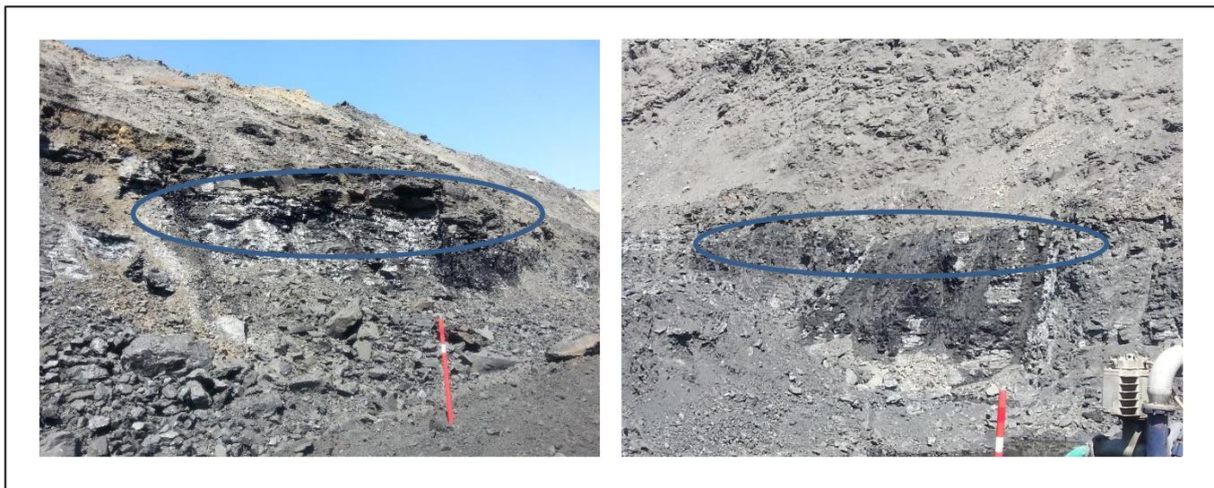
Figure 2.21: Lateral seepage flow from geological contact zone (bedding plane)
