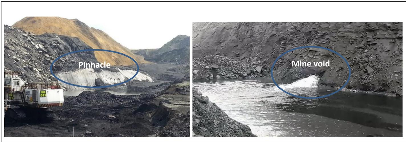
**Figure 2.23: Water accumulation in the vicinity of a pinnacle (doline structure) and water flowing out of the mine workings.**
