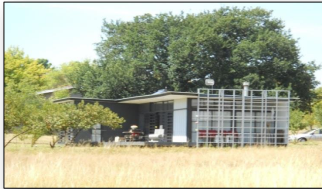
Figure 5.19 An example of a steel-frame house in Rosendal (Source: Visser)
