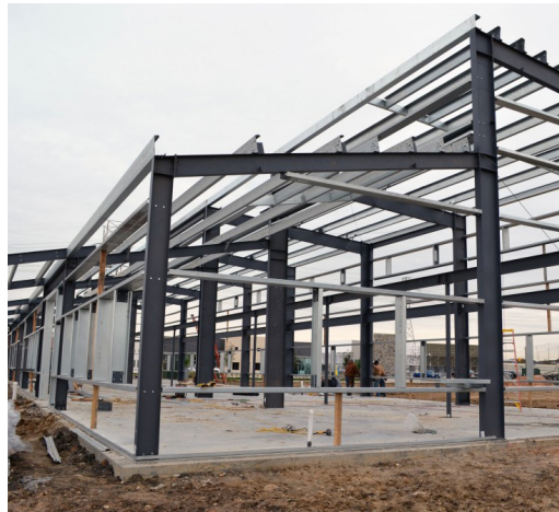
STEEL FRAMING [PRIMARY STRUCTURE]
