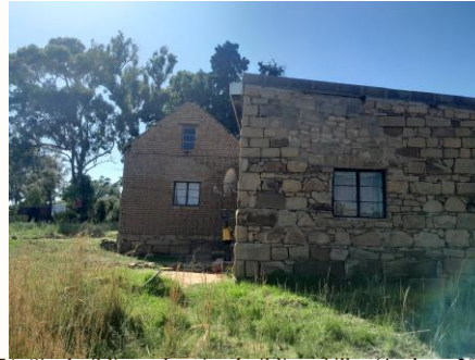
Fig. 174: Site buildings showing building skills. (Author, 2023 )
