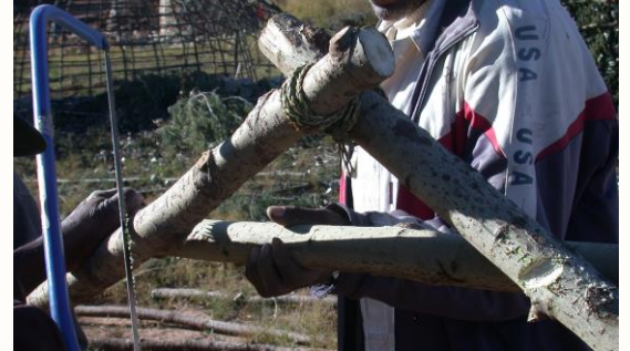
Fig. 156: Basotho men, making gum pole trusses at Thaba Bosiu (Khatleli, 2011 )
