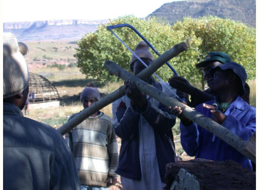
Fig: 147. Basotho men, making gum pole trusses at Thaba Bosiu (Khatleli, 2011 )
