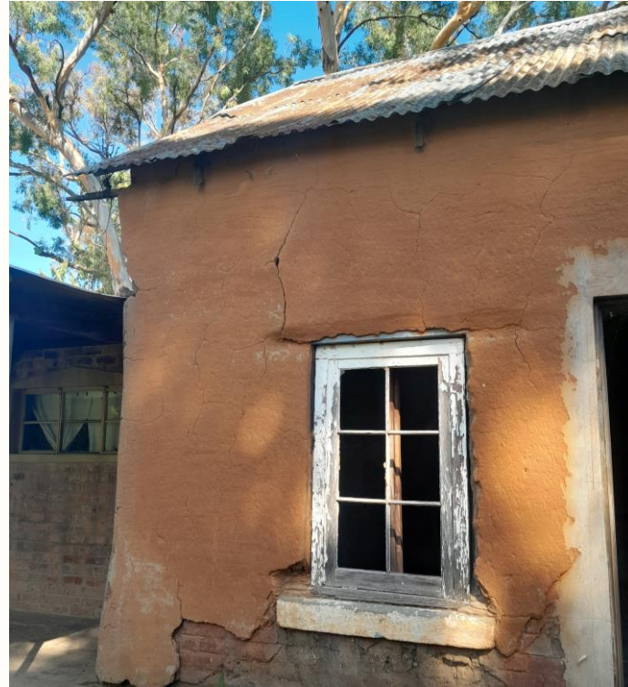
Fig.172: Site buildings . (Author, 2023 )
