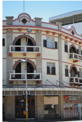
Fig.56+ Fig. 57: Existing corner details which are reflected in the new addition
