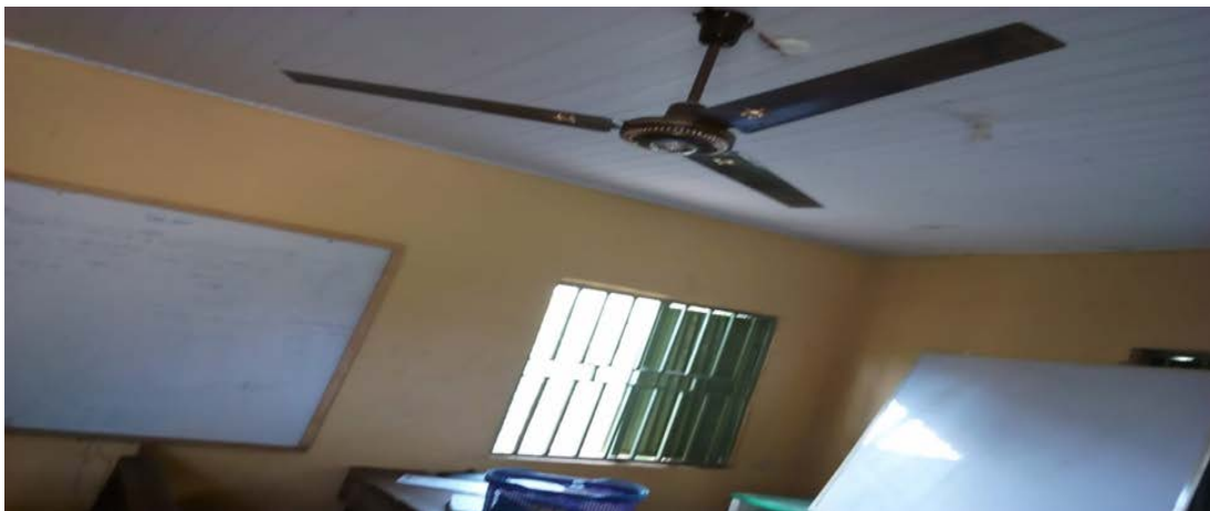
Figure 5.18: ICT building (inside view)
