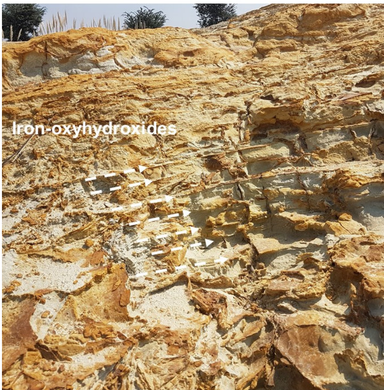
Figure 12: Exposed top 2 m of tailings dam showing parallel lamination/bedding as well as heavy mineral fractionation that resulted in iron-oxyhydroxide enriched laminae (July 2015).
