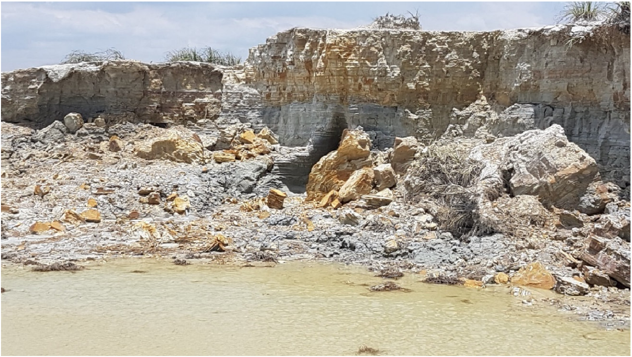
Figure 9: A newly exposed part of the tailings dam showing a distinct oxidised zone in the first 2-3 meters (October 2016).
