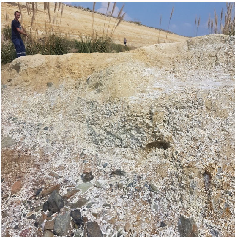
Figure 14: Secondary mineral precipitates from toe seepage. The photo was taken at the northeastern corner of the tailings dam (April 2017).
