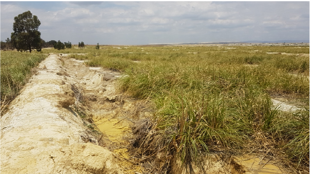
Figure 10: The surface of the tailings dam with overgrown paddocks and minimal water drainage (July 2015).
