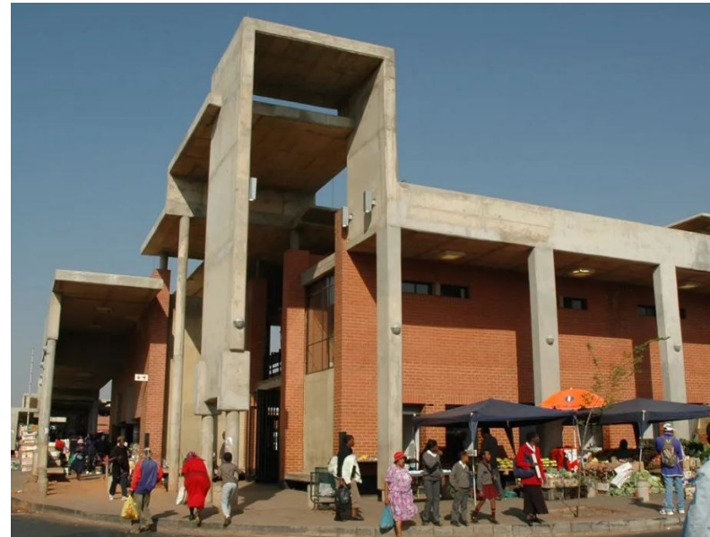
Figure 149: Vendor spaces along the side of the building promotes a sense of porosity (MATHENGE, 2015: online).
