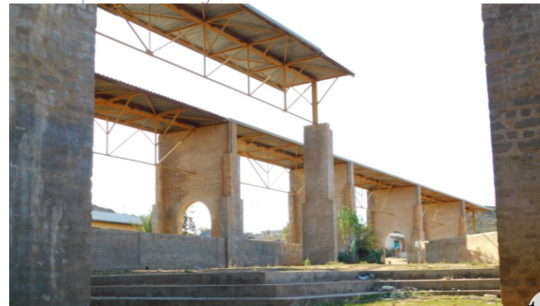
Figure 172: The porous colonnade of Steinkopf Community centre (author,2022).
