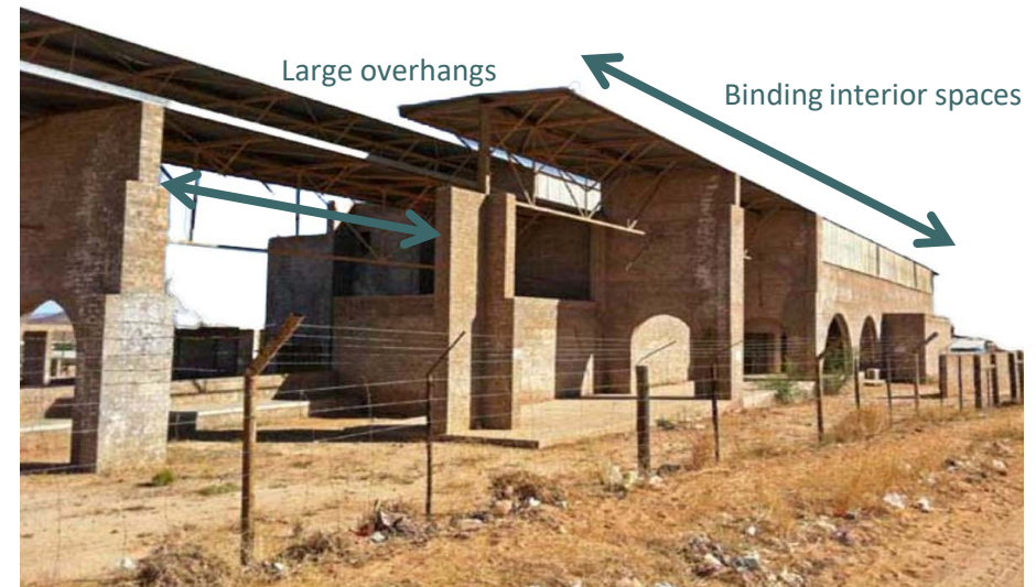
Figure 178: Roof spans large open areas, binding interior spaces and creating exterior circulation spaces (author, 2022).
