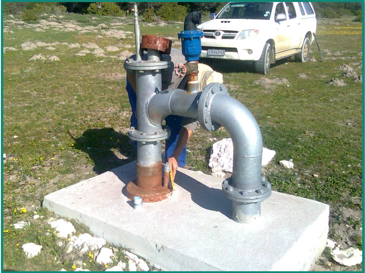
Maintenance at BG00136 (25 August 2010)
