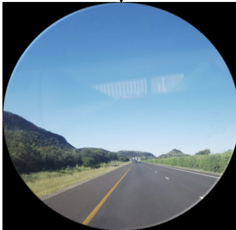
N1 Road passing site
