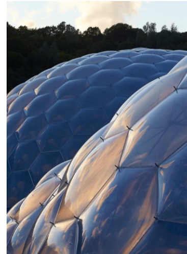
Figure 182 & 183: Detail of ETFE Pillows (Architen Landrell, 2013:2).
