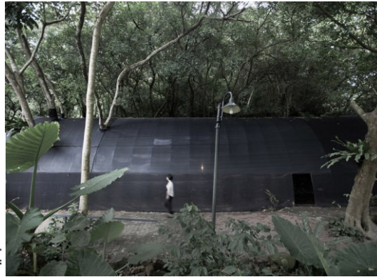
Figure 176: Exterior Façade (ArchDaily, 2014: online).
