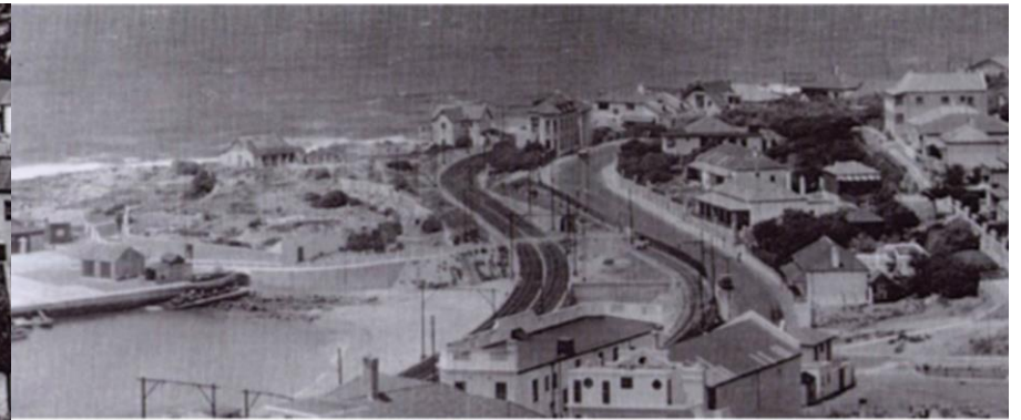
Figure 2.11: The Point in 1933: fish plant, powerhouse and cottagers demolished; "Patmos" demolished; "stable" remodelled; "By-the-Sea" rebuilt to a double storey; railway doubled (Gasson, 2002: online).
