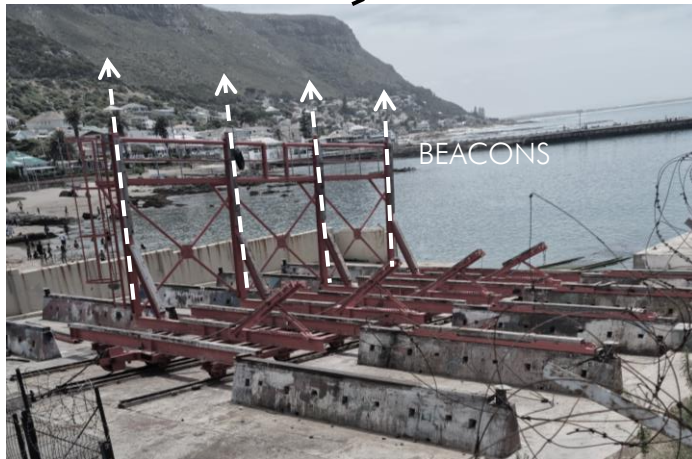
Figure 2.38: Beacons on site (Author, 2022).
