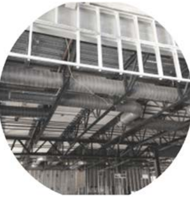
Fig 4.3.BP: Acoustic roof installation (Brooke, 2014: online)
