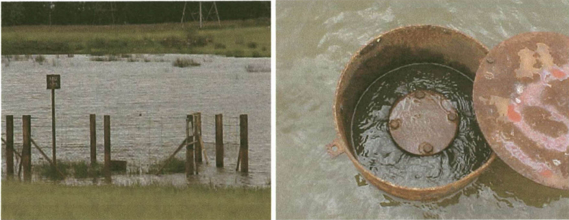
Figure 65. Dam with surface run-off and recharge borehole from the dam into the mine
