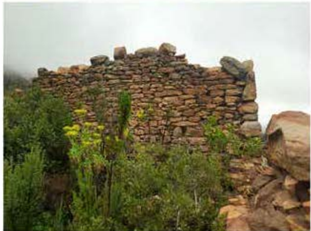
Figure 194-195: Use of stone stacking building techniques to build structures along pass while building pass (author, 2020)
