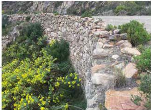
Figure 196: Use of stone stacking building techniques to build pass (author, 2020)
