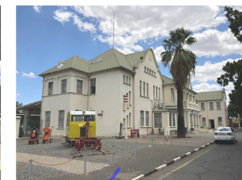
Existing station entrance
