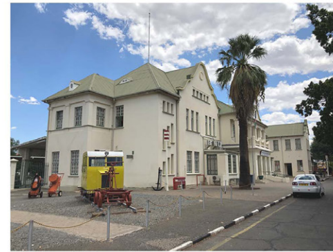
Existing station entrance
