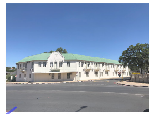
Existing underutilised building completed in 1930
