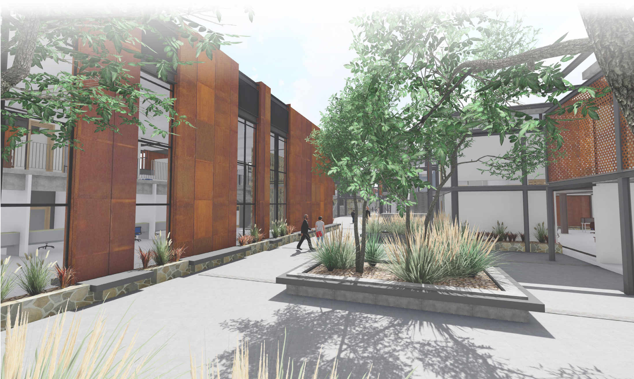
CENTRAN COURTYARD OF LONG-DISTANCE BUS STATION (left) & 4X4 RENTAL (right)
