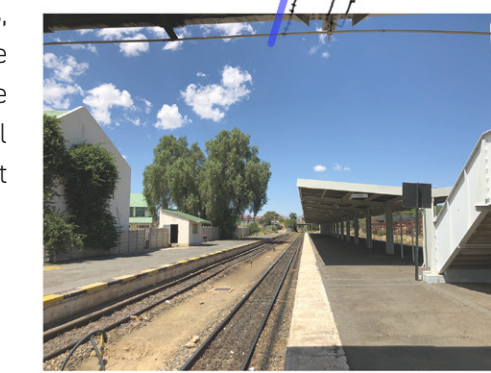
Existing railway platforms
