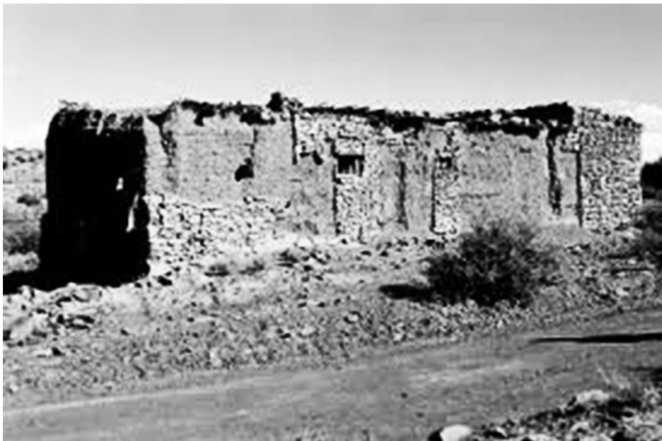
Figure 96 - Vernacular earth brick house (Maguire, 2004)
