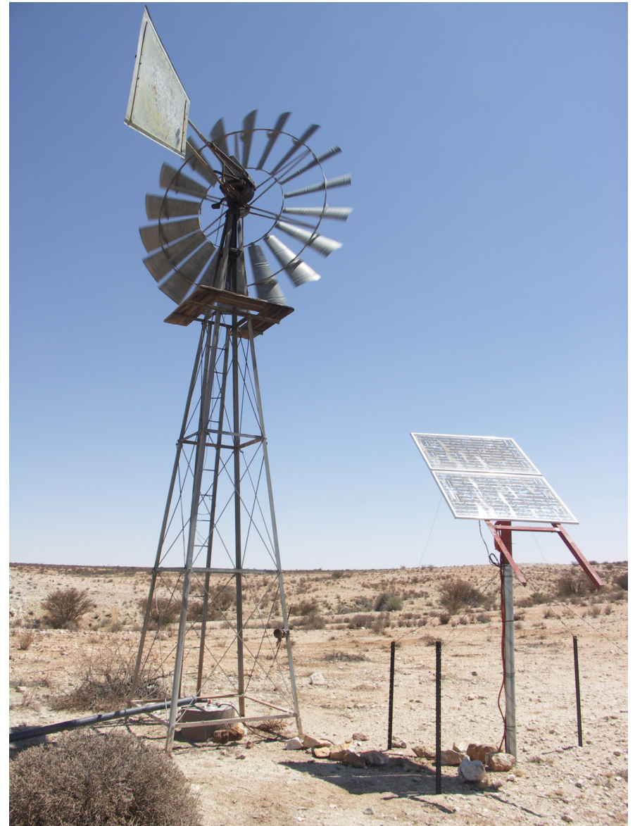
Figure 98 - Solar pump replacing windpump, (solarpumps.com, online)
