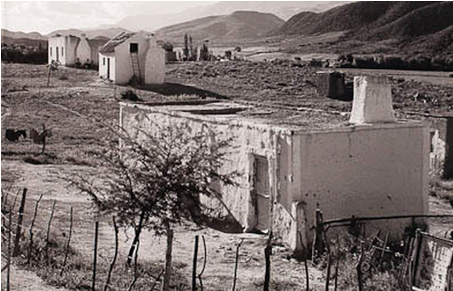
Figure 113 - Brakdak roof (Fagan, 2008)
