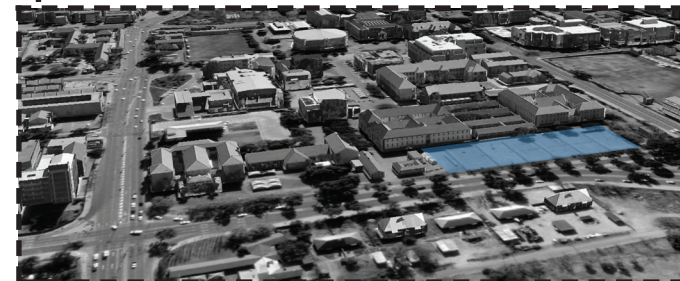
Figure 05 Aerial View of Site taken from Google Earth,2019.
