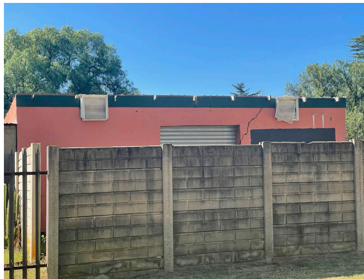
Figure 48: Refer to 4,5,6 on location layout: Smallholdings next to Everett on Vaal (Author, 2022)
