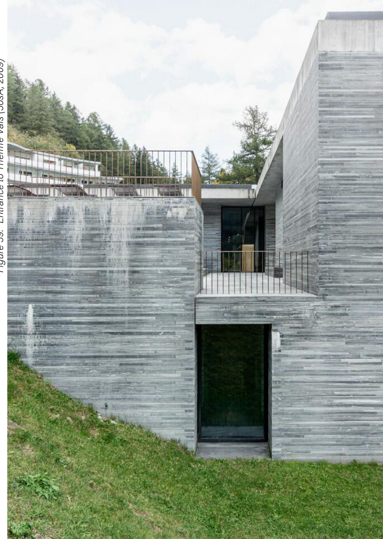
Figure 59: Entrance to Therme Vals (5osA, 2009)
