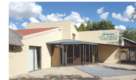
Figure 33: Brandwag Islamic Centre (Author, 2021).
