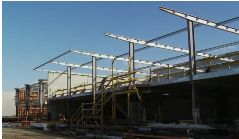
Figure 169: Superstructure of the accommodation and service block (wocomoCULTURE, 2021: online).
