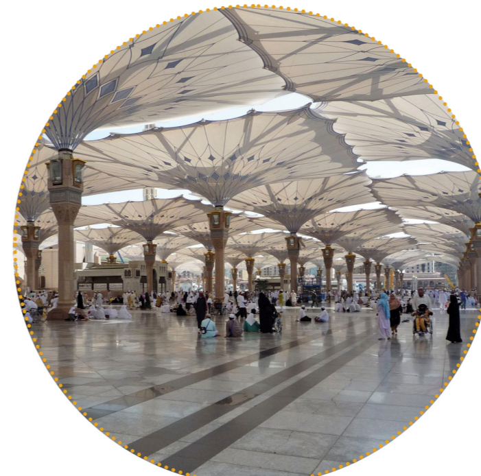
Figure 182: Mechanical umbrellas used in the courtyard at the Prophet's Mosque in Medina (Abdullatif Al Fouzan Award, 2011: online).
