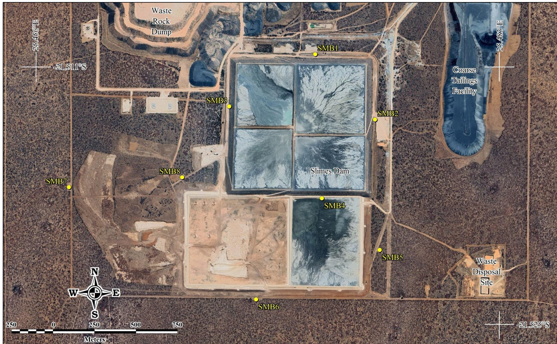
Figure 4.21: Monitoring boreholes for the slimes dam.
