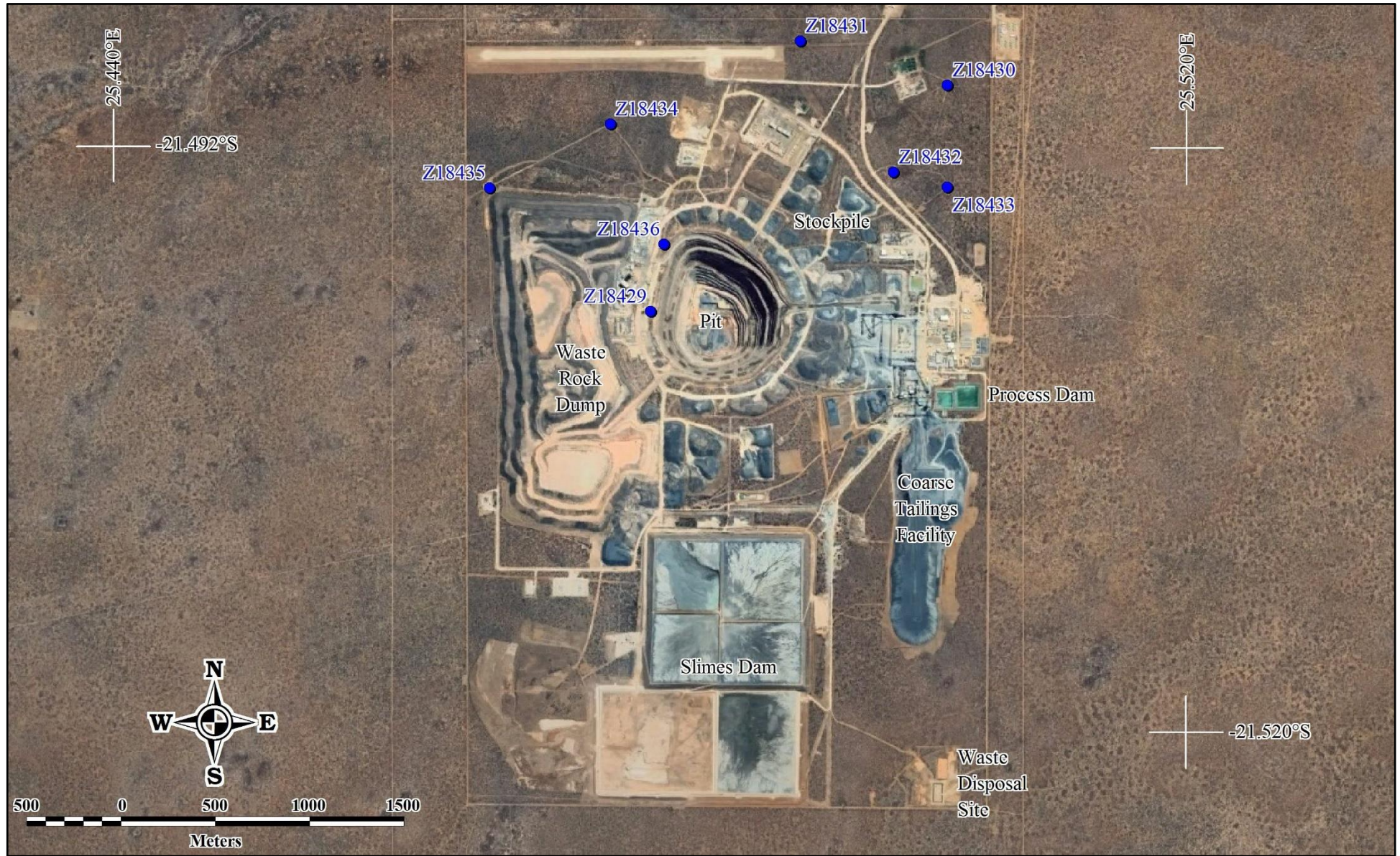
Figure 4.2: Positions of the wellfield boreholes at KDM.
