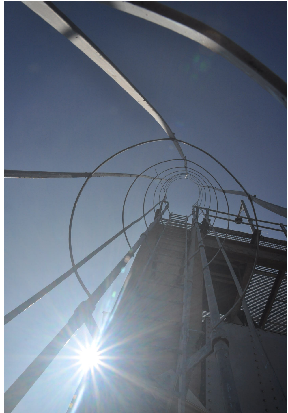
FIGURE 13: Ladder to the top of the dam (Author, 2023).
