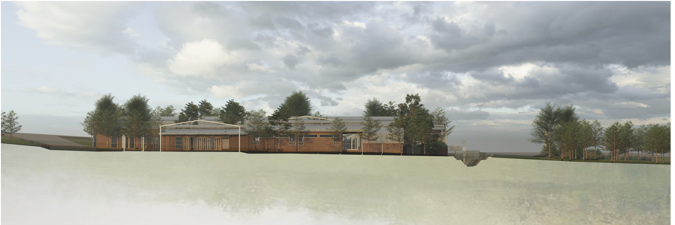
FIGURE 297: North-Eastern Elevation (Author, 2023).
