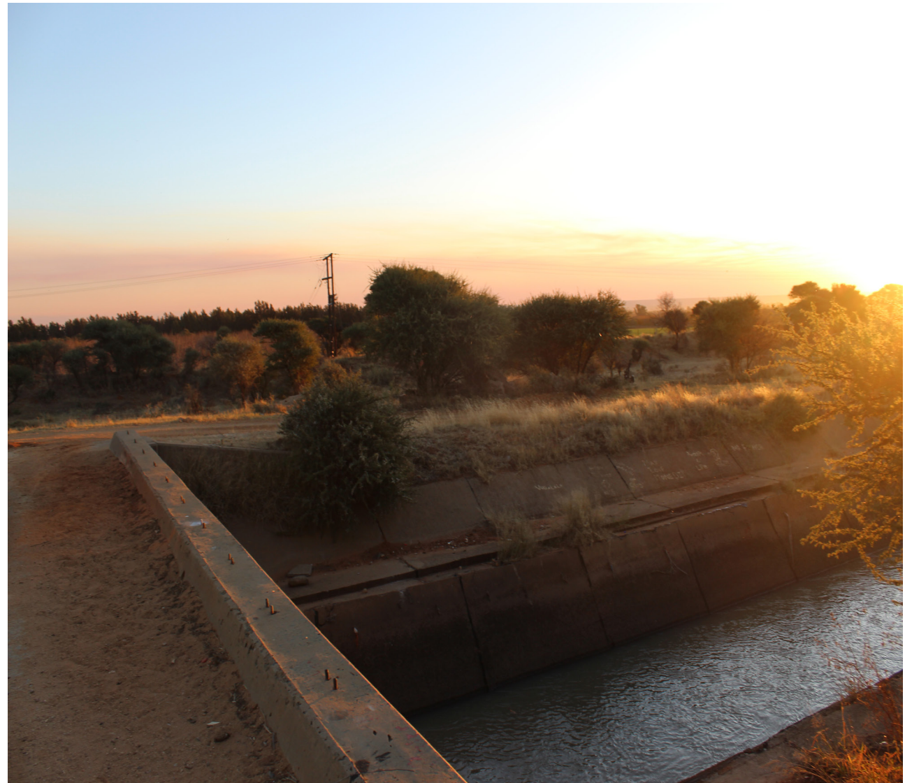
FIGURE 68: Photo of site showing the canal, road and bridge (Author, 2023).
