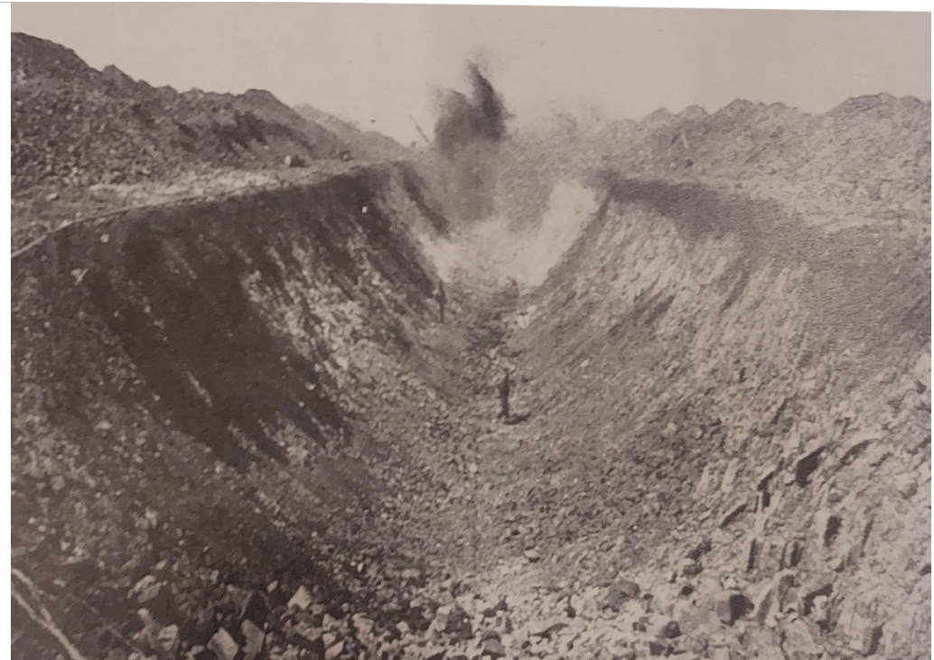
FIGURE 45: Dig site for the canal (van Rensburg, 1935).
