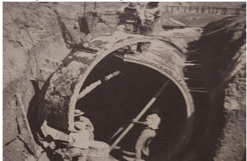
FIGURE 46: Construction of the Northern tunnel (Botes, 1937).
