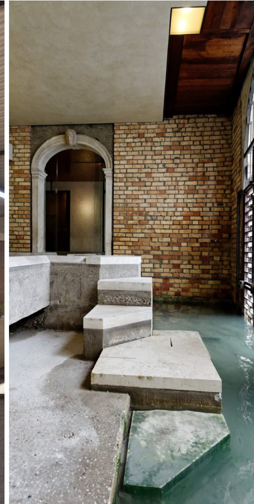
FIGURE 316: Renovation at water gates (de Cal, 2019).
