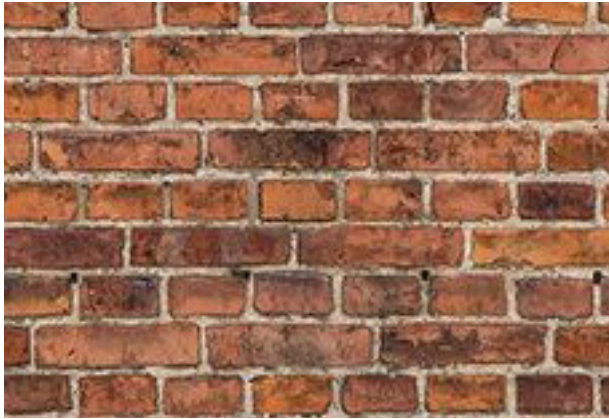
FIGURE 342: Exposed brick surface (Brick Cladding, 2022).
