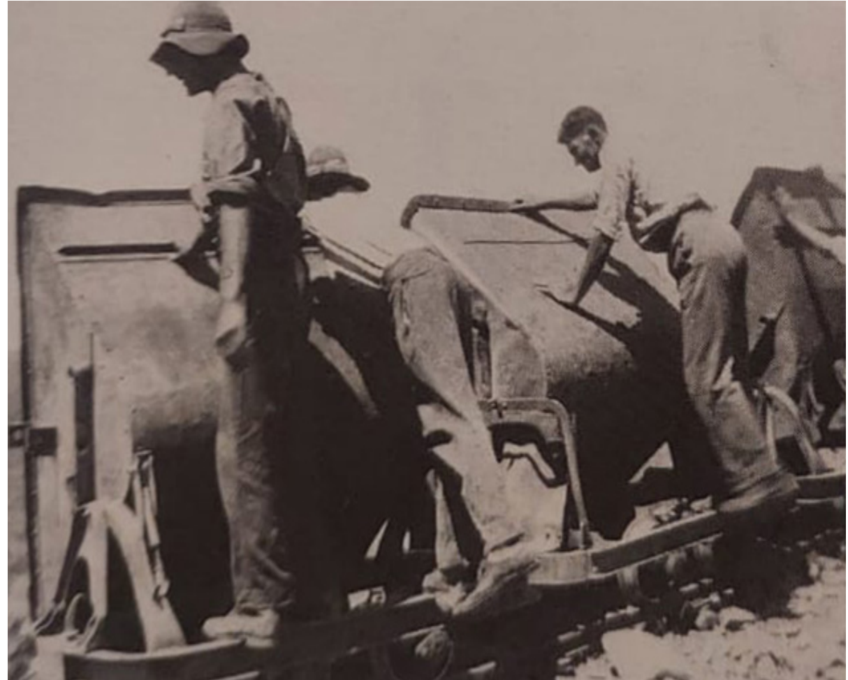
FIGURE 33: The mixing of cement, to cast the floor base of the canal (Botes, 1937).
