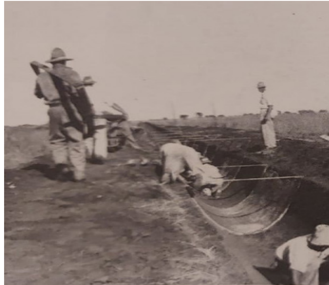
FIGURE 36: Process of building the separation canals captured in photo (Botes, 1937).
