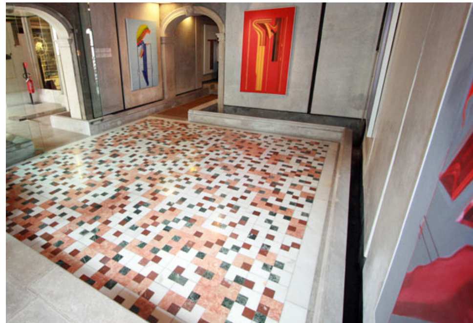
FIGURE 317: Renovation at groundfloor (de Cal, 2019).
