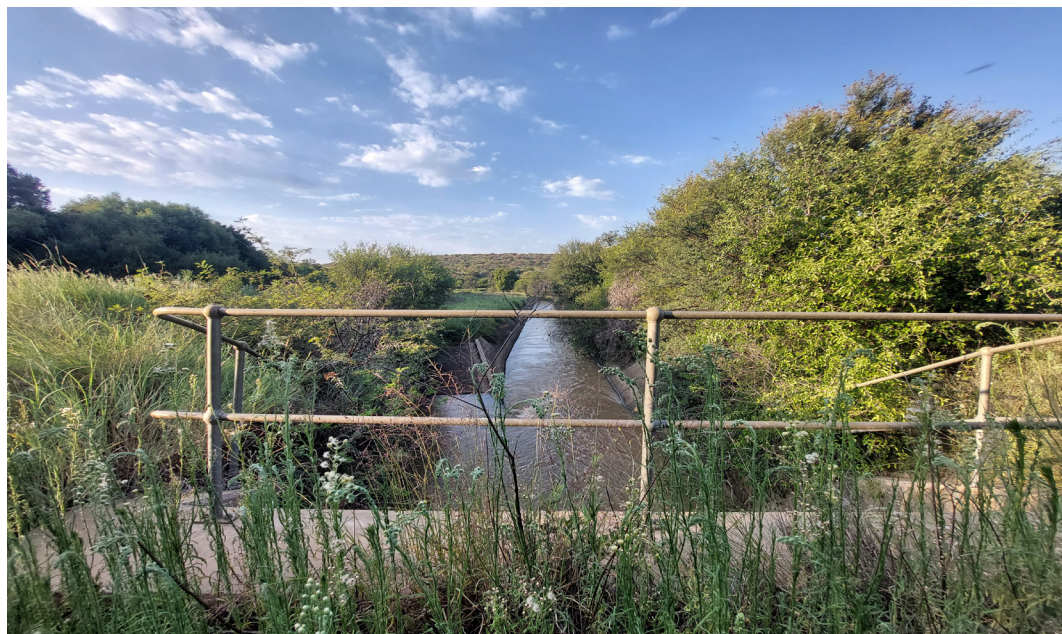
FIGURE 38: Outlet of the Southern tunnel through the hill (Author, 2023).
