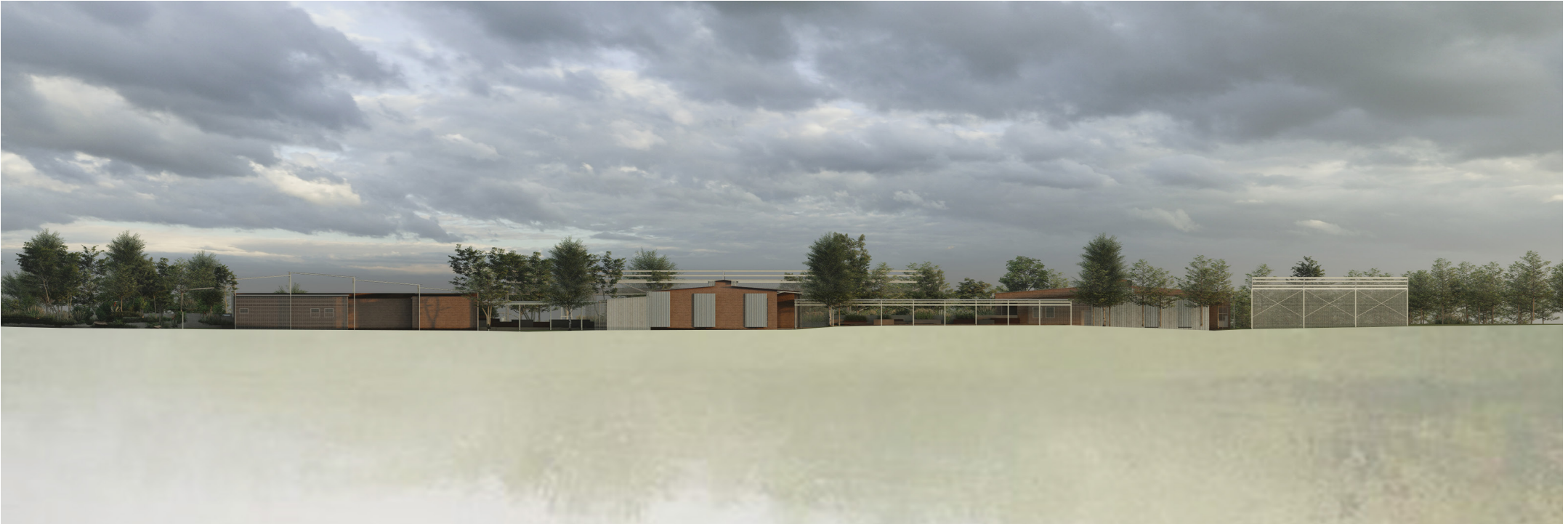
FIGURE 299: North-Eastern Elevation (Author, 2023).
