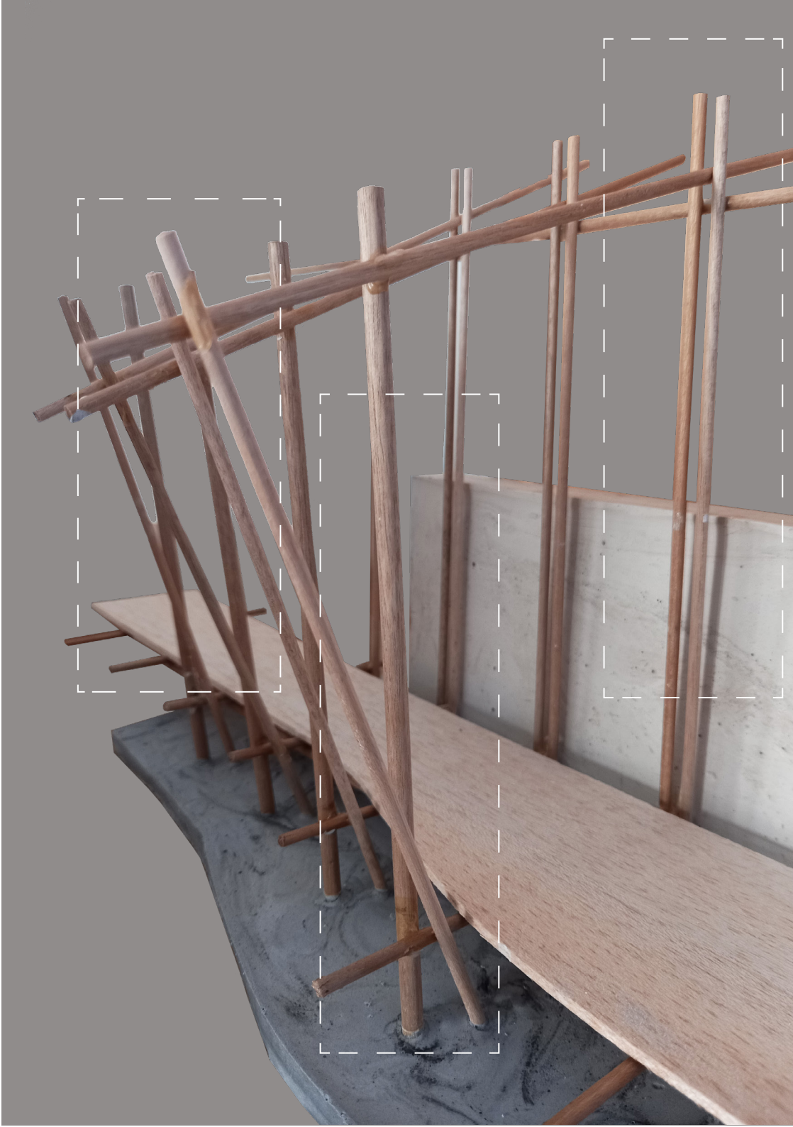
Figure 1: Post in drilled hole on land (Author. 2023)
