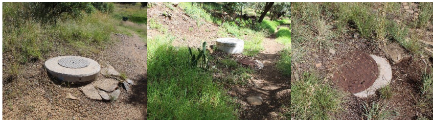
Figure 40 - Scattered man-holes over site and 7 Dams conservancy.
