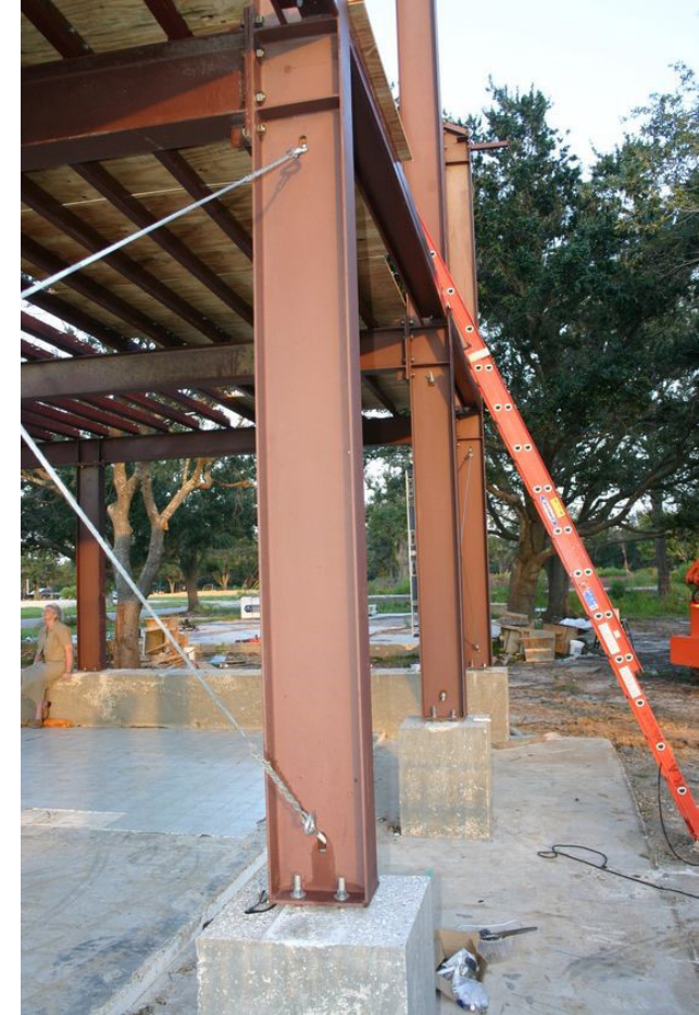
Figure 68 - Steel raised structure (R. Wood, 2009)
