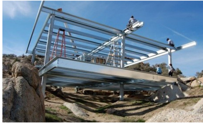
Figure 67 - Lightweight Steel framed structure molding into the rocky outcrops (Jetson Green, 2009)
