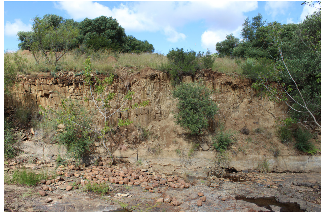
Figure 50 - Excavated soil on the higher rocky hills, showing the ground make-up. (2019, P. Vorster)
