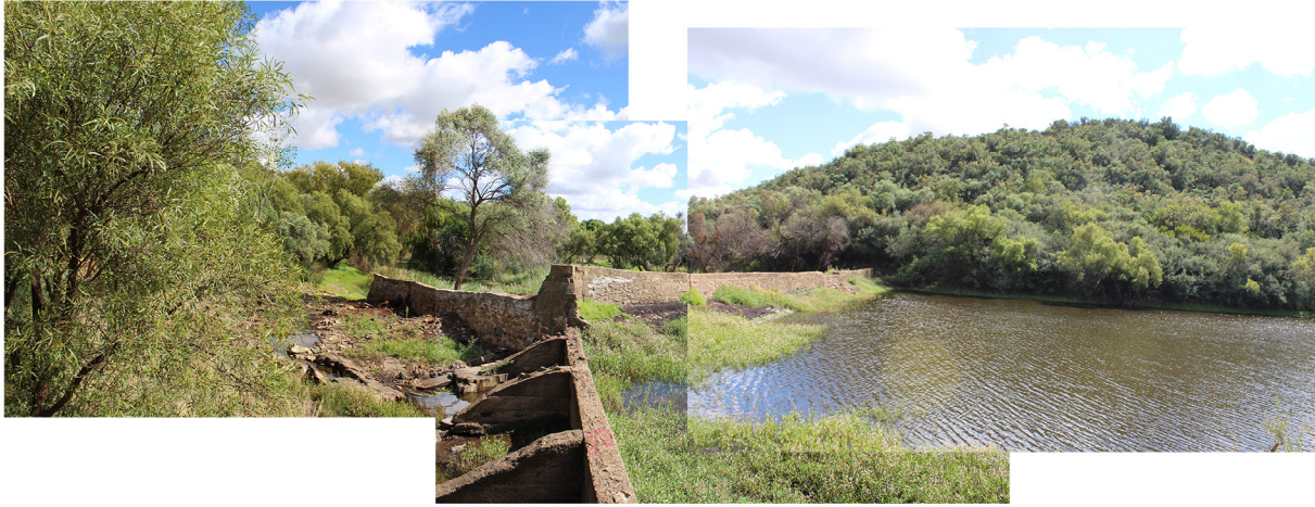
EXISTING DAM WALL
