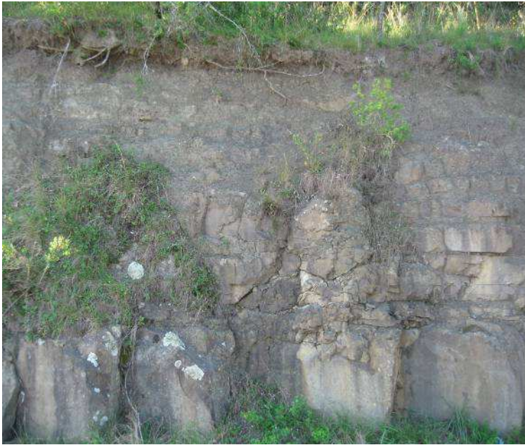
Figure 5.6 Shrubs and trees growing in the bare rock with cracks near catchment B3.
