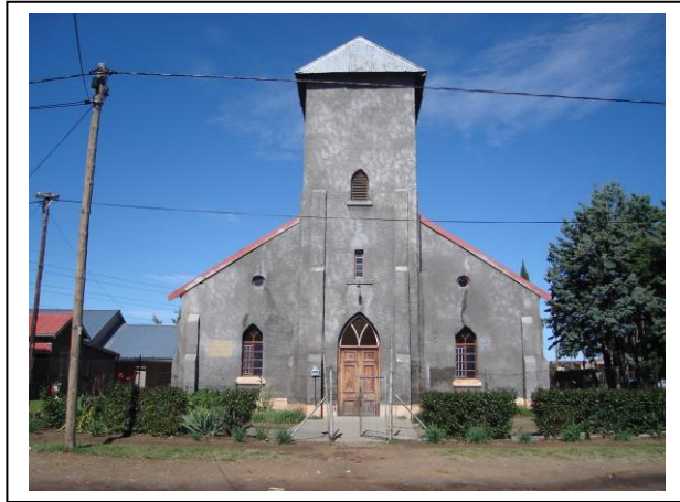
Image 5/17: AME Church, Gonyane Street, Batho, circa 2010. Note remnants of clipped hedges in front of church (National Museum: NM Photo Batho 144)
