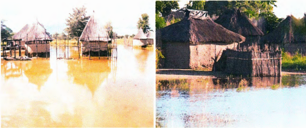
Figure 3.4 Waterlogged Villages in the Zambezi region soon after heavy rainfalls resulted in flash flooding
