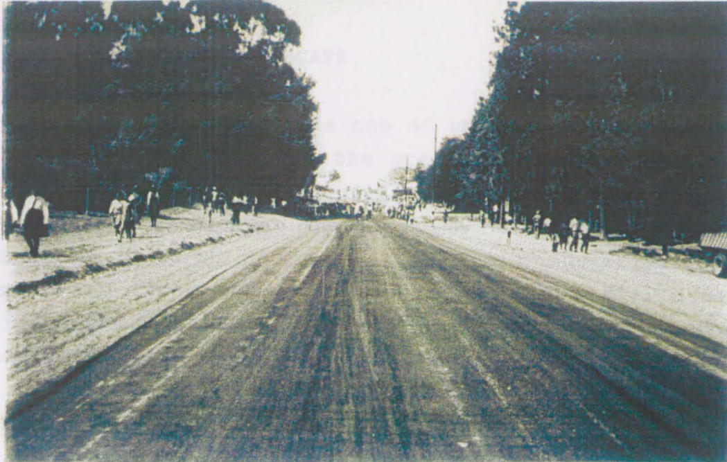
PHOTOMAP 5.6 THE PRE-INDEPENDENT (Above) AND THE INDEPENDENT INFRASTRUCTURAL DEVELOPMENT (Below) THE CONTRAST LIES IN THE TARRED STREETS, ELECTRICITY, AND STORM WATER DRAINAGE
