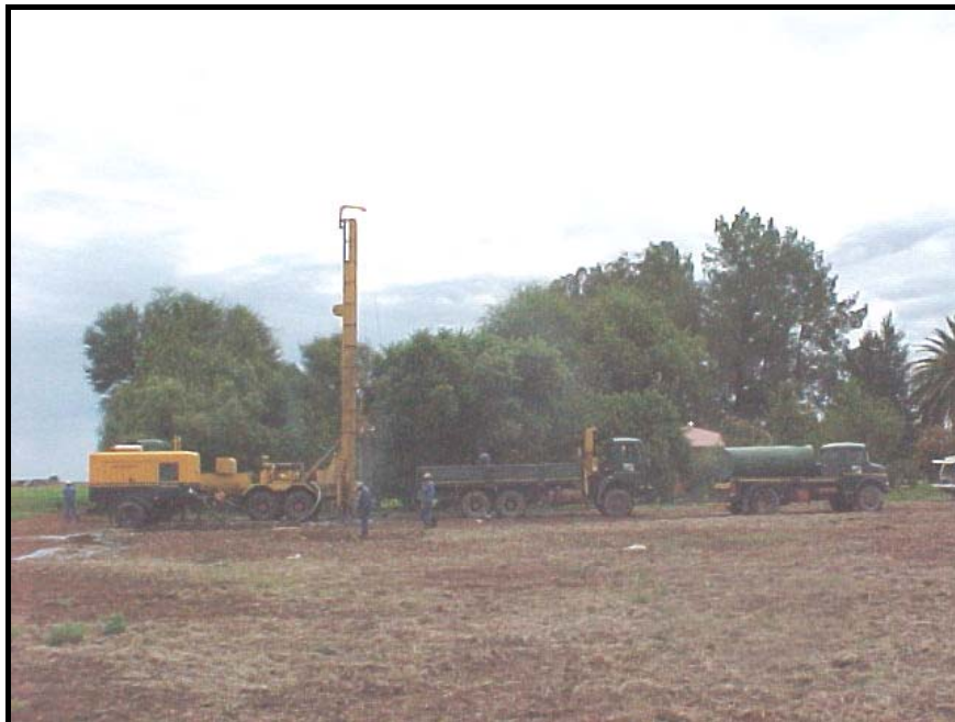
Figure 22:DWAF drilling rig and support vehicles used in the Vaalharts project
