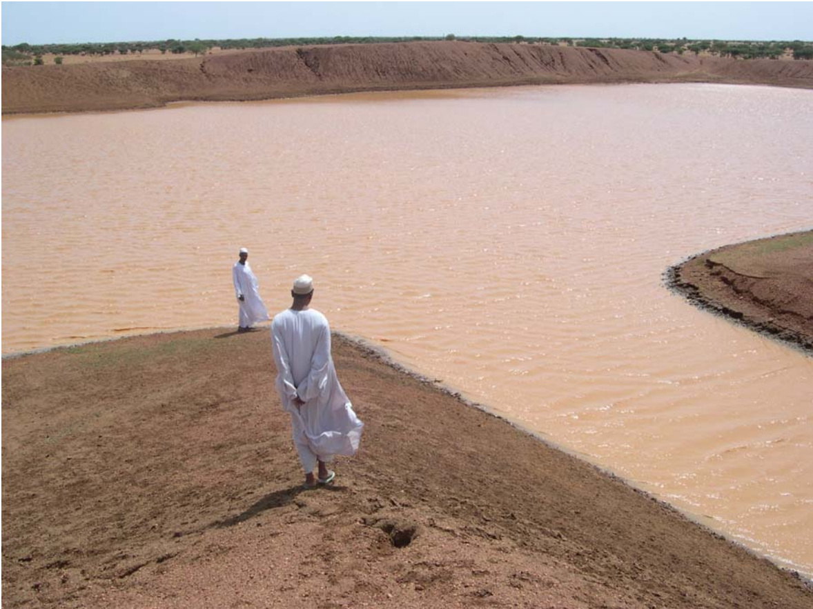
Plate 5.2 Hafir with store of rainfall water during the field survey to ElKhatow village (photo courtesy S. Walker, August 2005)
