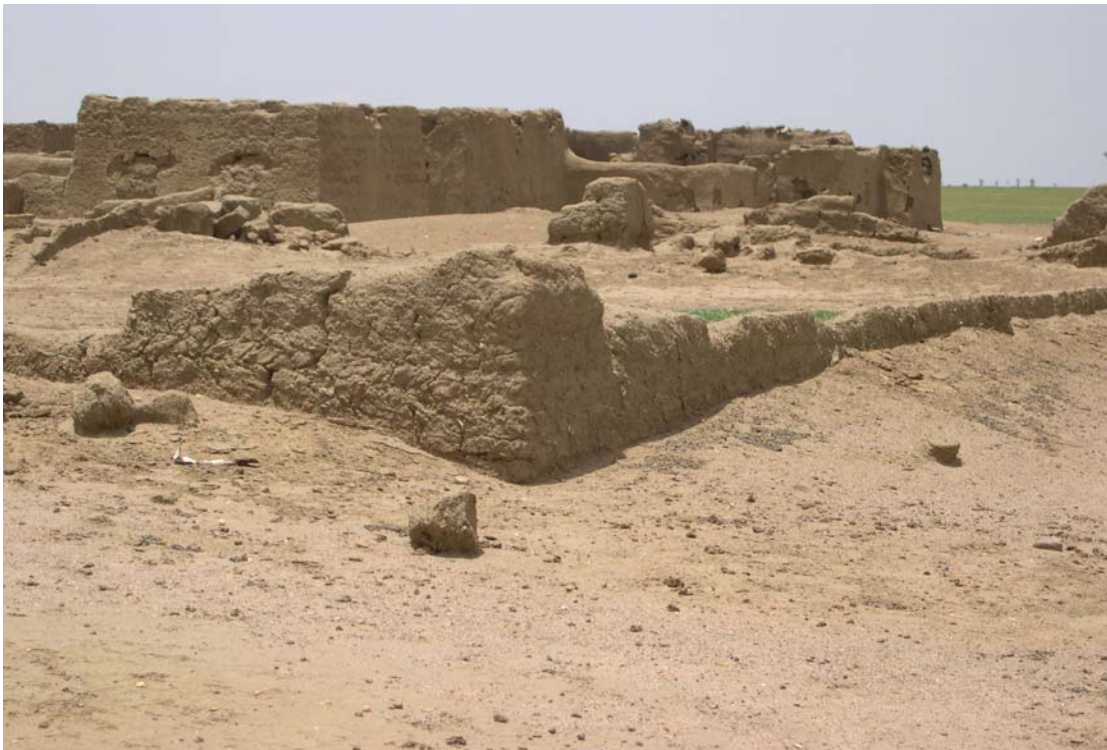
Plate 4.3 Houses in Shakia Mekkia village that were completed washed away by water erosion after a rain event in August 2005 (photo courtesy S. Walker, August 2005)
