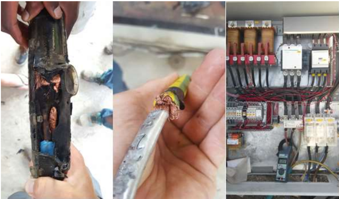
Figure 6-5 Photographs depicting a shorted cable joint due to incorrectly sized ferrules and crude crimping. The image on the far right depicts the replacement transformer (impedance) panel used after the soft starter panels were damaged.
