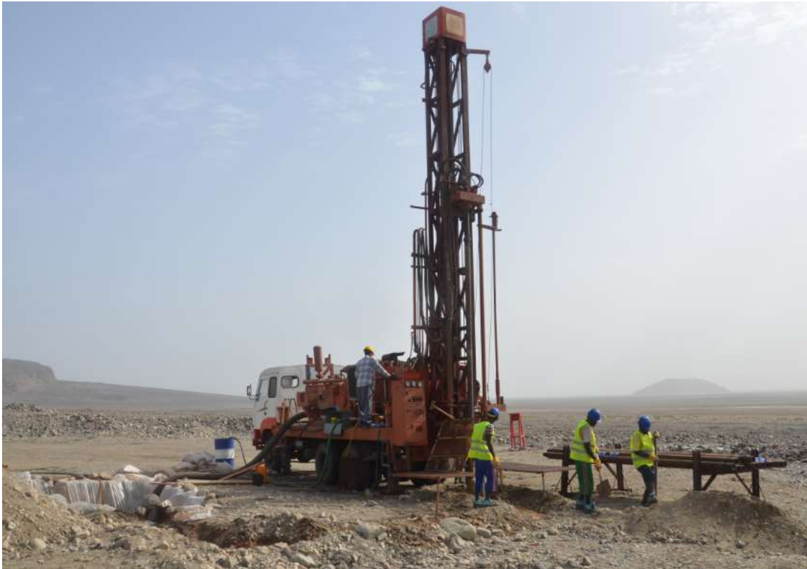
Figure 5-1 Mud rotary drilling technique. Shown is the smaller KLR rig drilling at DN-M02.
