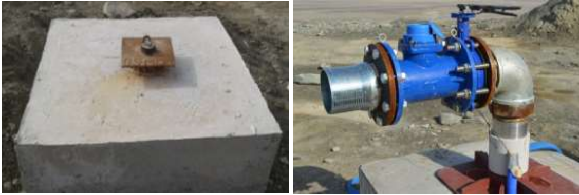
Figure 5-11 Final well head construction at BS-M01 and BS-P01.
