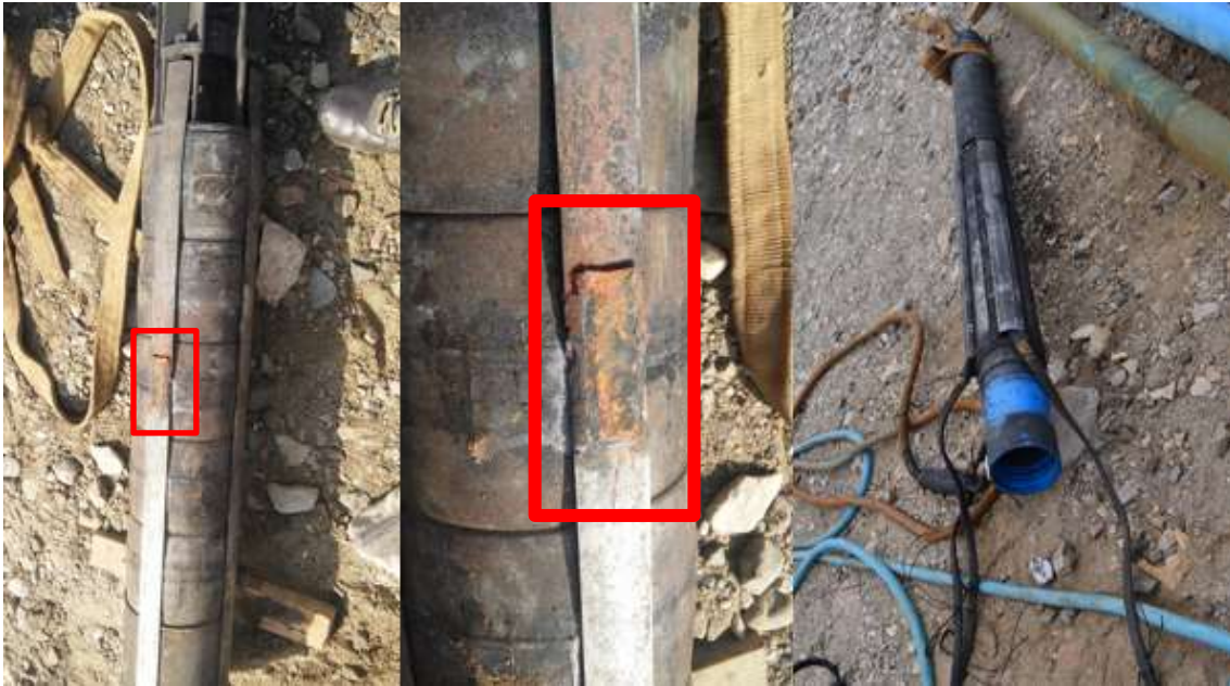
Figure 6-4 Photograph of the Grundfos pumps installed in RAJ-1 and RAJ-2. Corrosion to the tie rod and pump housing is evident.
