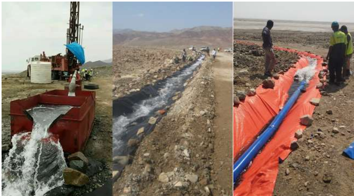
Figure 6-1 Photographs illustrating the V-notch used to measure discharge and the plastic lined trench that transmitted water down the fan to prevent recirculation during pumping.
