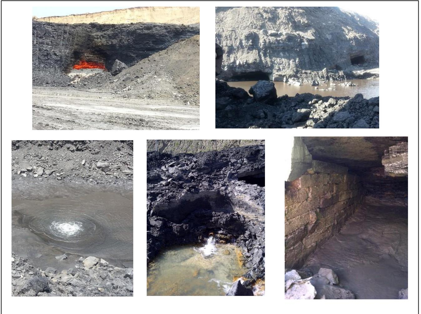
Figure 2.22: Photos of different areas of the old mine workings showing areas that are dry, filled with water and an area with a constructed compartment wall.
