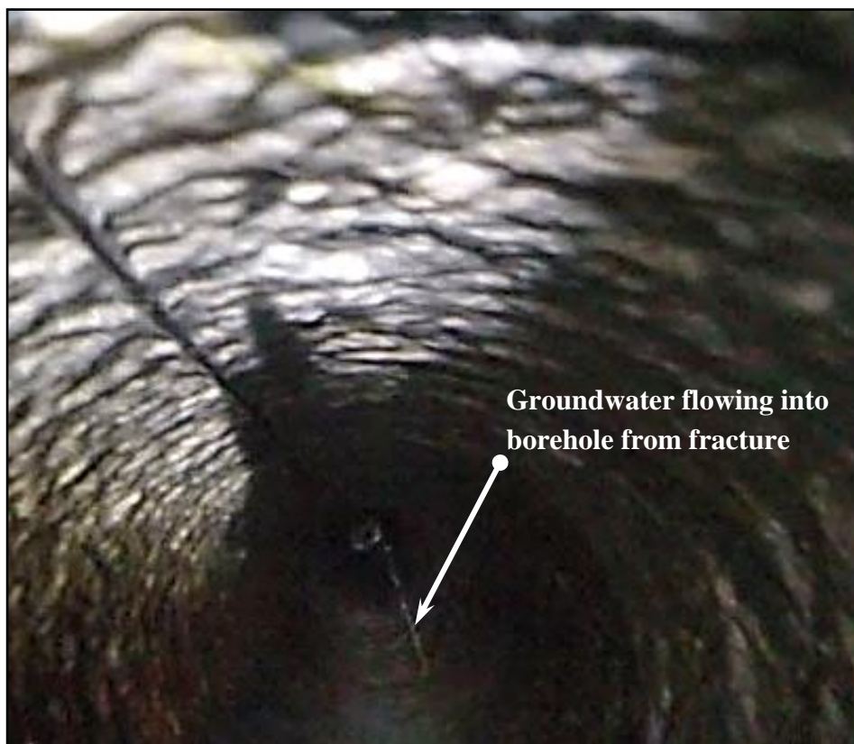
Figure 5.45 Fracture at 43 m (LR004A).
