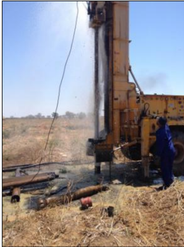
Appendix A-3: An example of a water strike at LF004A.
