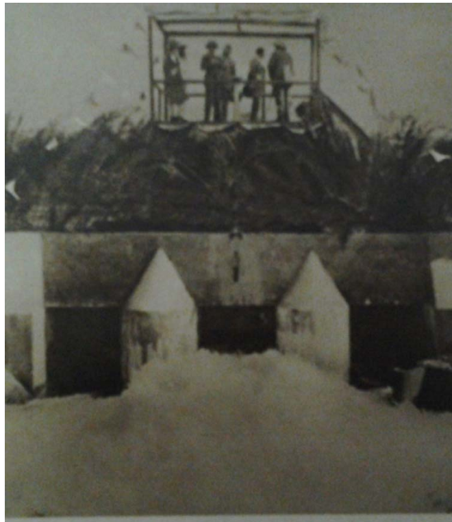
OPENING THE MULUNGUSHI HYDRO-ELECTRIC POWER SCHEME- BROKEN HILL 1925
