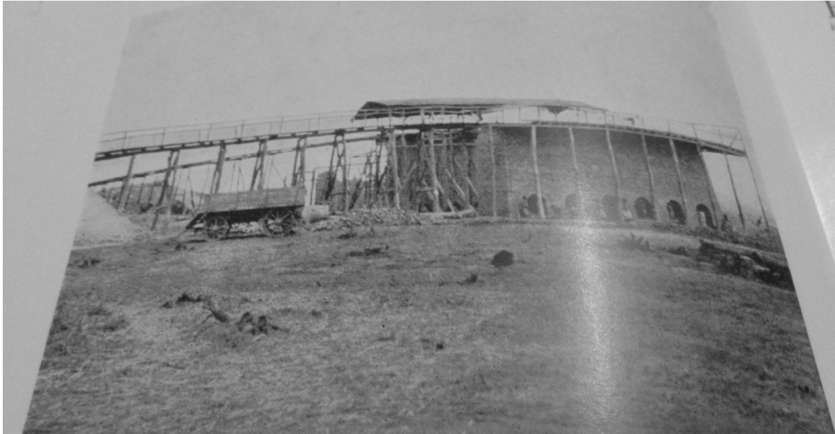
Figure 1: A SIDE VIEW OF THE FIRST FURNACE TO BE CONSTRUCTED AT BROKEN HILL
