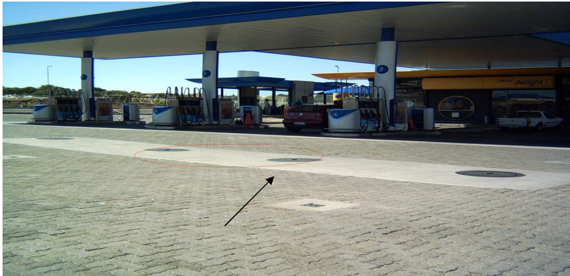
Photo 7.1: Example of monitoring wells
