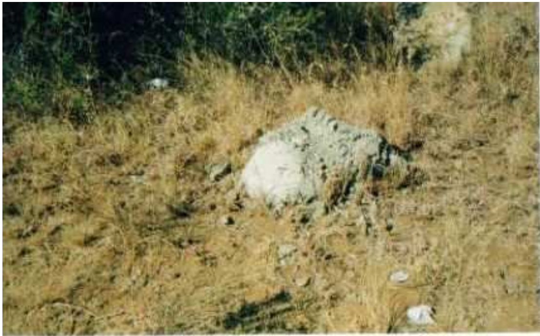
Photo 10: Example of concrete residue on soil
