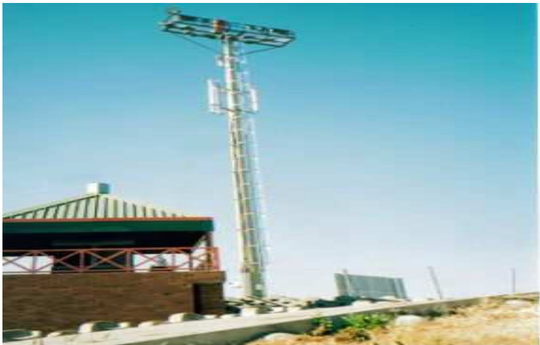
Photo 5.5: Example of a floodlight used as a cell phone mast
