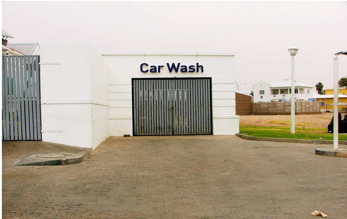
Photo 9.3.1: Example 3 of an unauthorised change to construction plans
