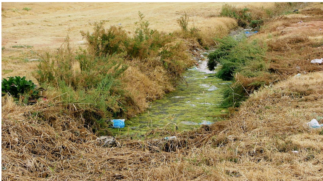
Photo 9.3.6: Storm water channel
