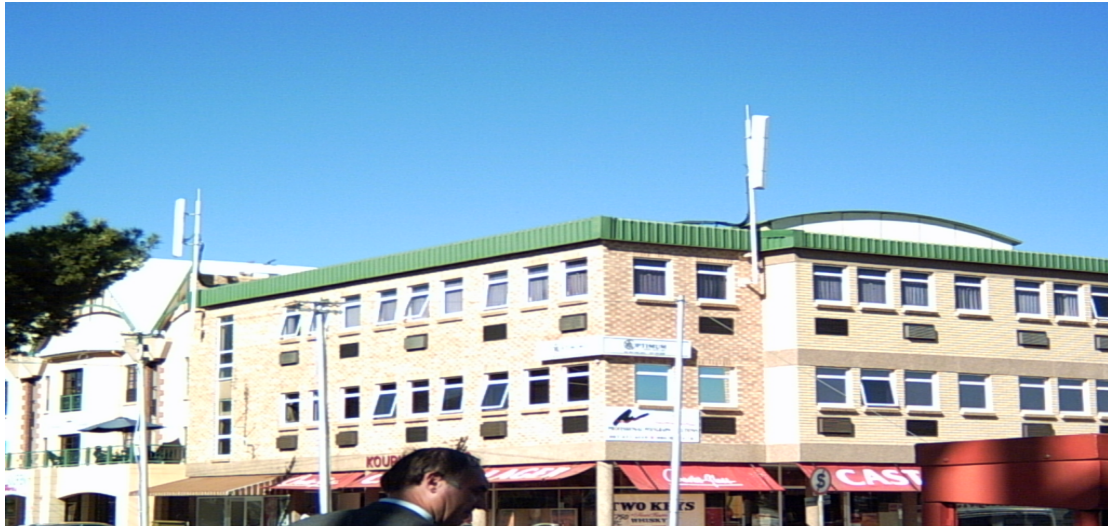
Photo 5.8: Example of rooftop antennas
