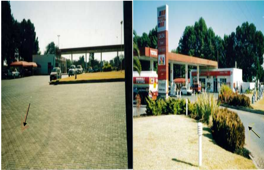
Photo 11: Example of the layout of a filling station
