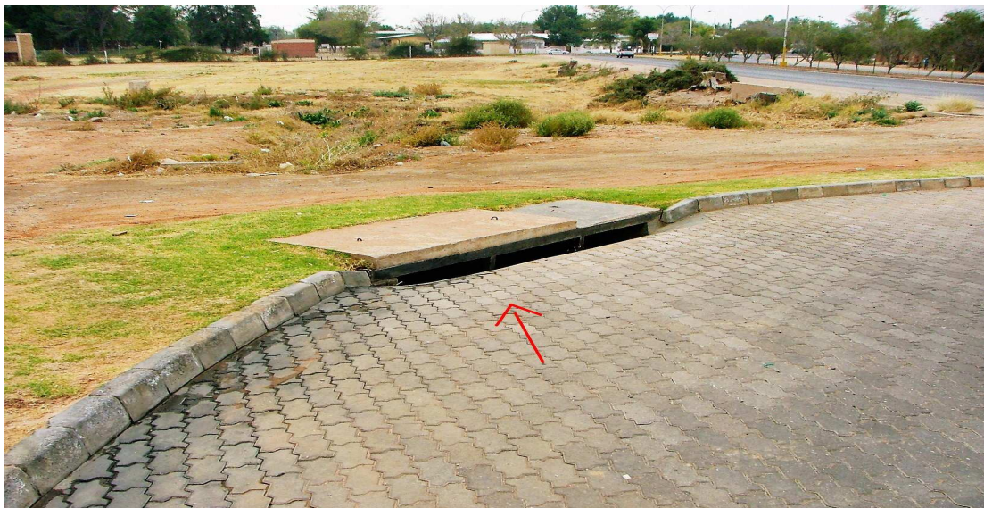
Photo 9.3.4: Storm water drain at filling station
