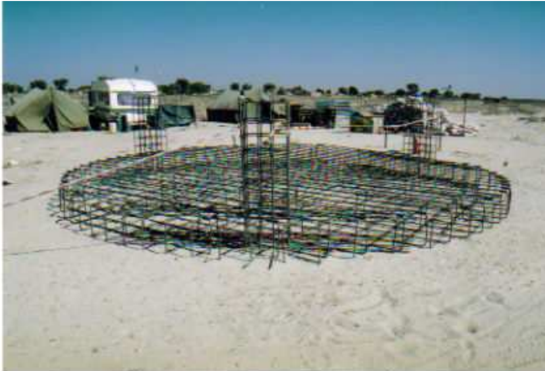
Photo 8: Example of a construction camp
