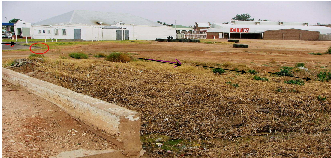
Photo 9.3.5: Flow from storm water drain
