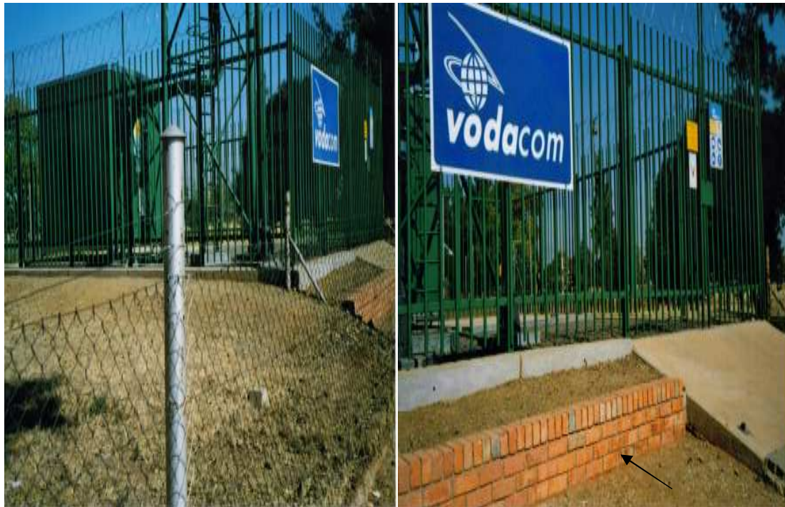
Photo 3: Example of a mitigation measure to prevent soil erosion
