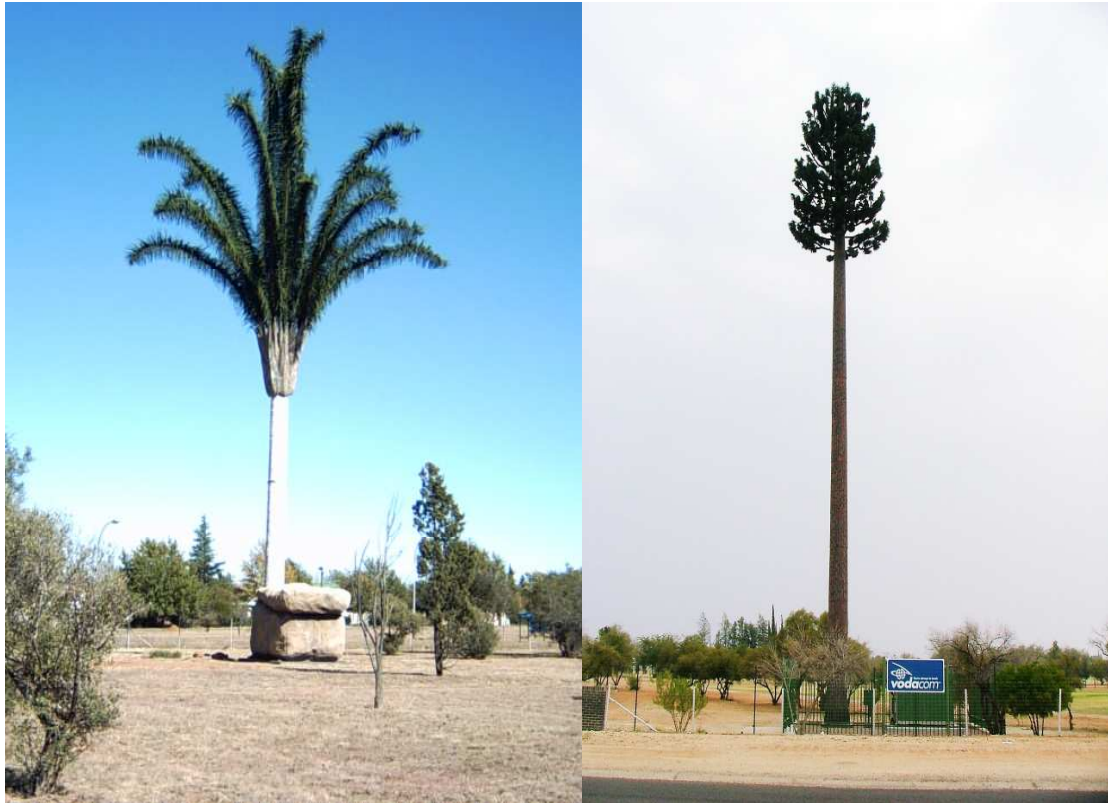
Photo 5.6: Example of Camouflaged masts
