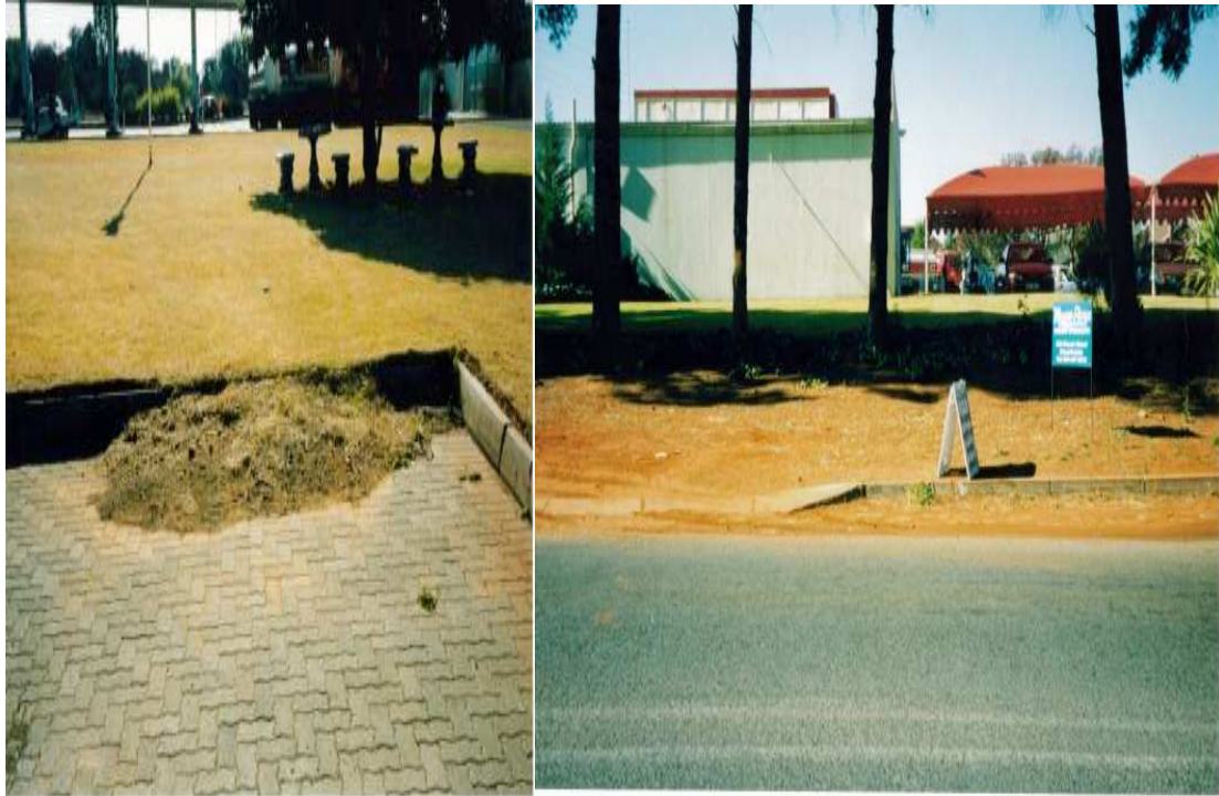
Photo 12: Example of inadequately implemented mitigation measures
