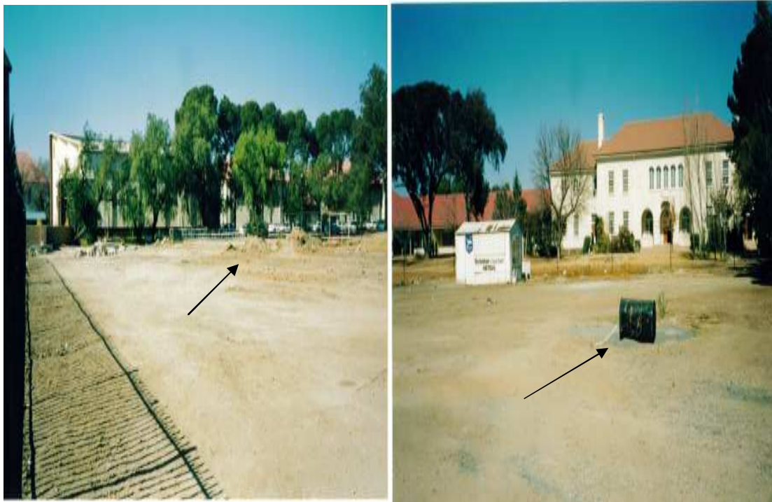
Photo 1: Example of construction waste not removed
