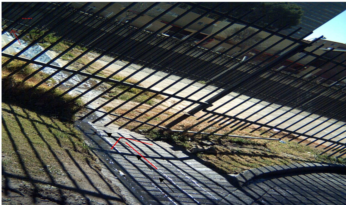
Photo 9.2.2: Runoff from car wash
