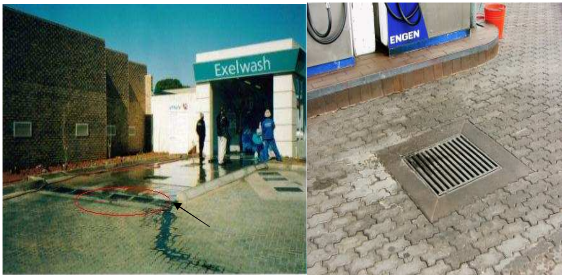
Photo 7.2: Example of oil interceptors
