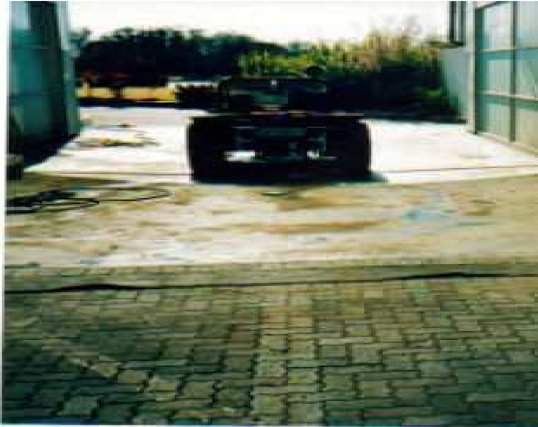
Photo 9.1: Example 1 of an unauthorised change to construction plans
