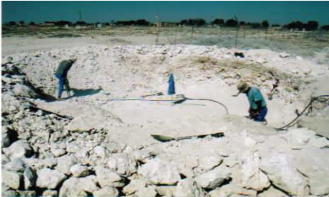
Photo 6: Example of earthworks
