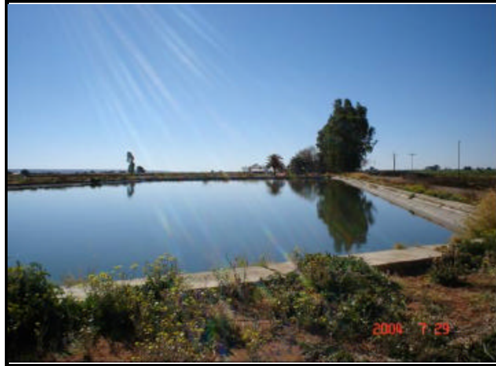
Figure 1. A typical irrigation dam in the Vaalharts Irrigation Scheme.
