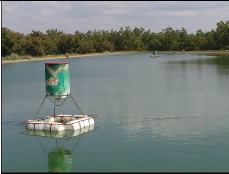
Figure 2. A photo of the screen preventing fish from escaping through the inlet of the irrigation dam in the Vaalharts Irrigation Scheme.
