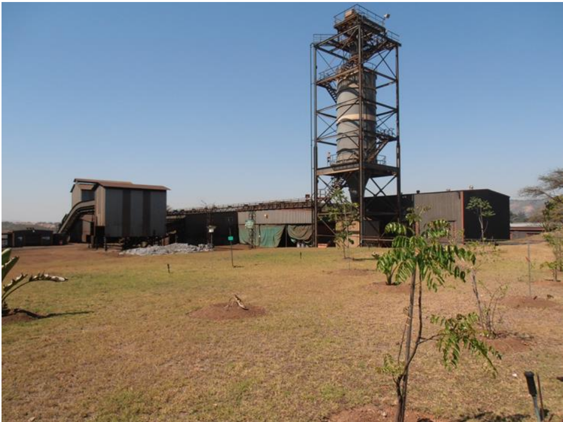
Figure 3-4: Delta E.M.D. facility near waste processing area looking towards the north east
