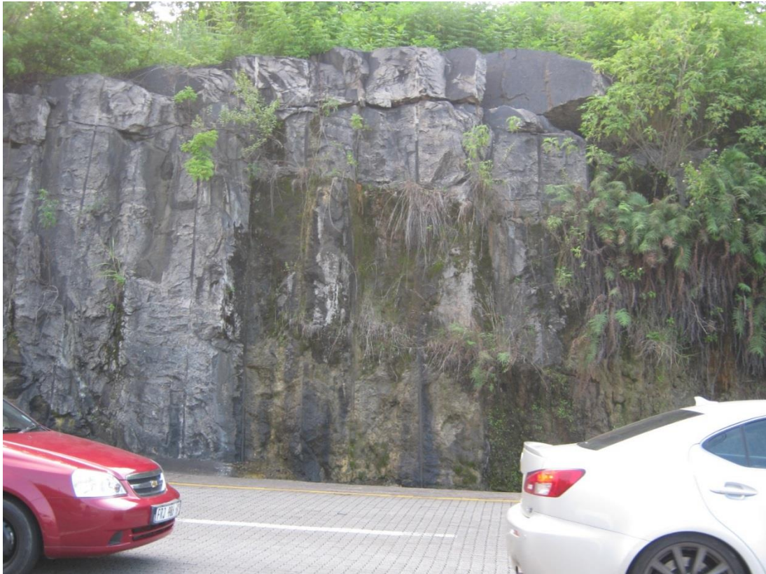
Figure 3-14: Shallow Water Seepage through Rock face to the west of the site
