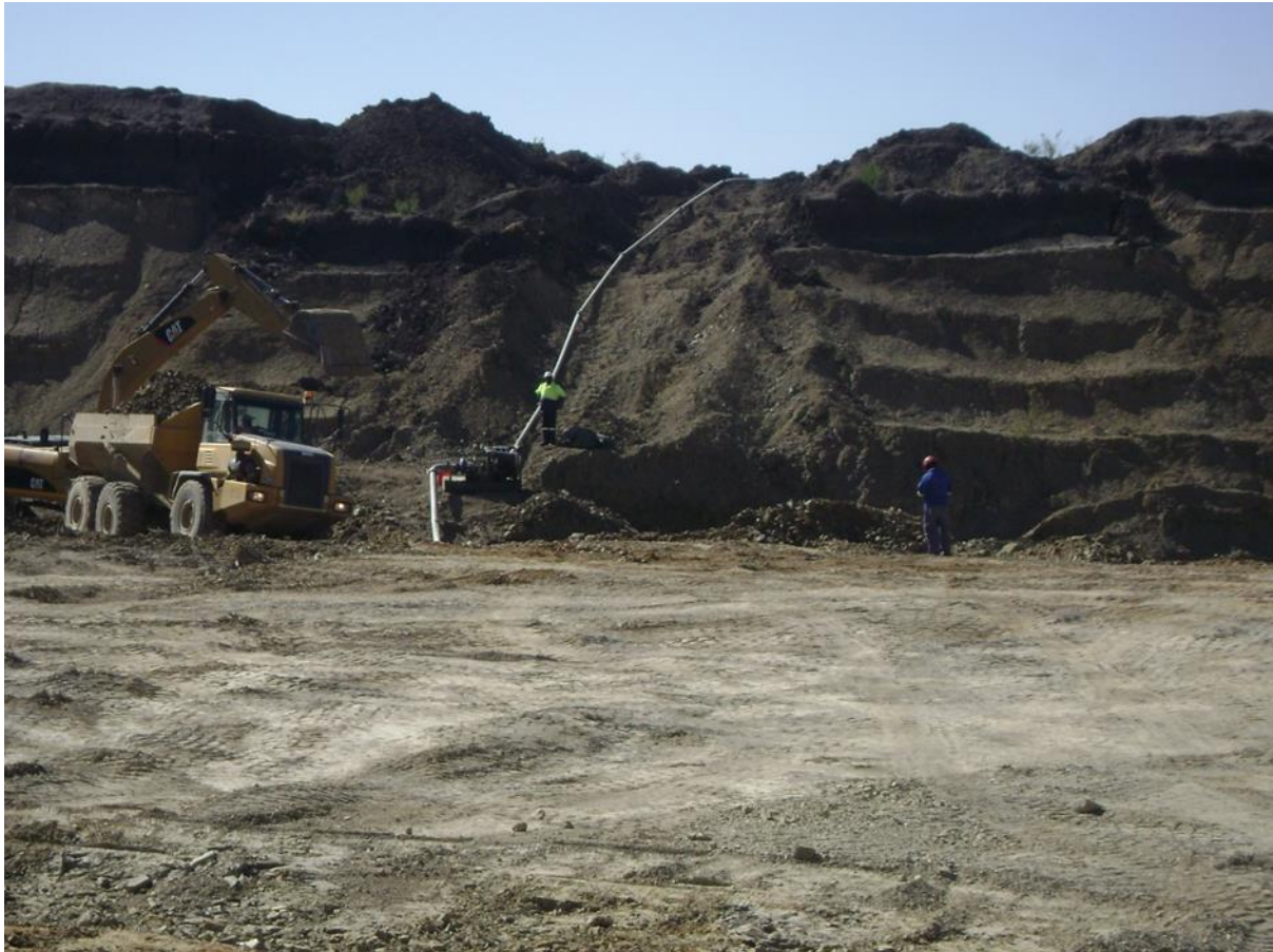
Figure 7-11: Dewatering of the pit at Matsopa Mine
