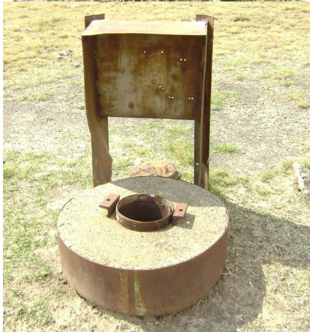
Figure 4-9: BH11 that is in use (top) and borehole that is no longer in use (bottom) at Ludwig farm
