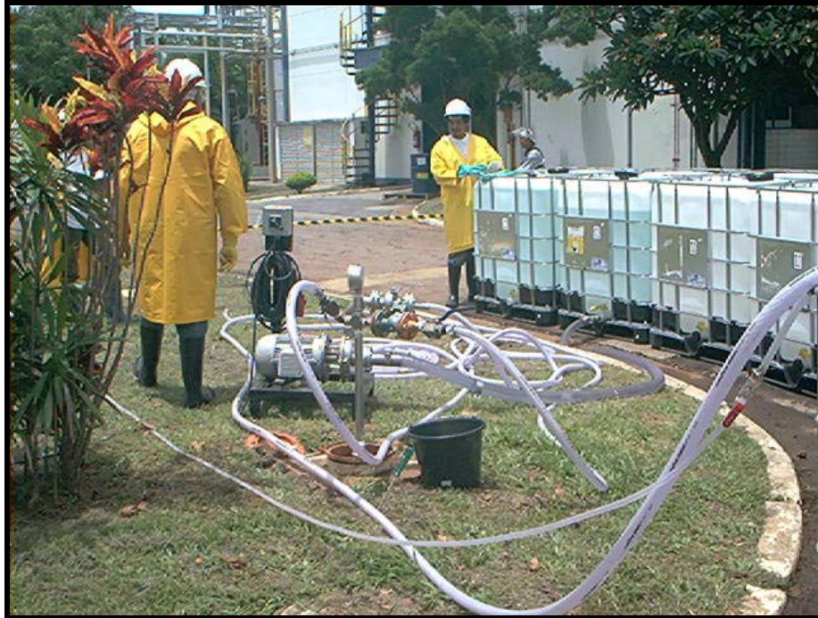
Figure 4.1 - Peroxide injection in the injection borehole PI-01, May 2003.
