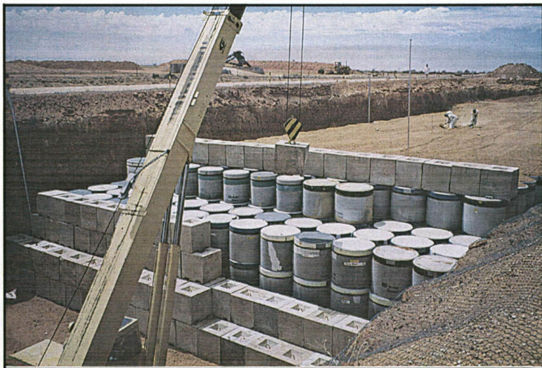
Figure 5-4 Near-surface earth trenches used for the disposal of low- and intermediate level waste at Vaalputs.
