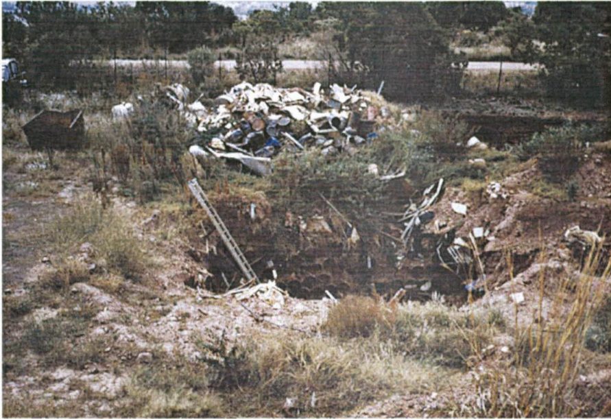
Figure 5-5 An excavated portion of Trench 7 at Thabana, which reflect a typical past practice near-surface disposal concept.
